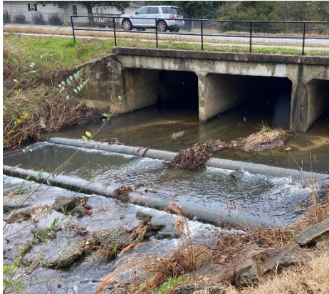
Example utility crossing at Gentilly Canal.
