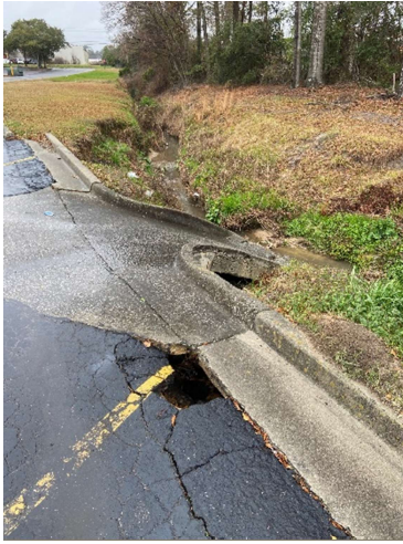
Compromised hydrologic structure.
