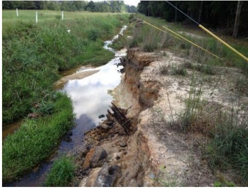
Drainage canal with severe erosion along the bank
