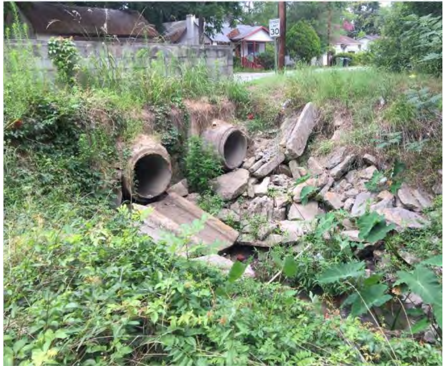
Headwall and existing pipes under road.
