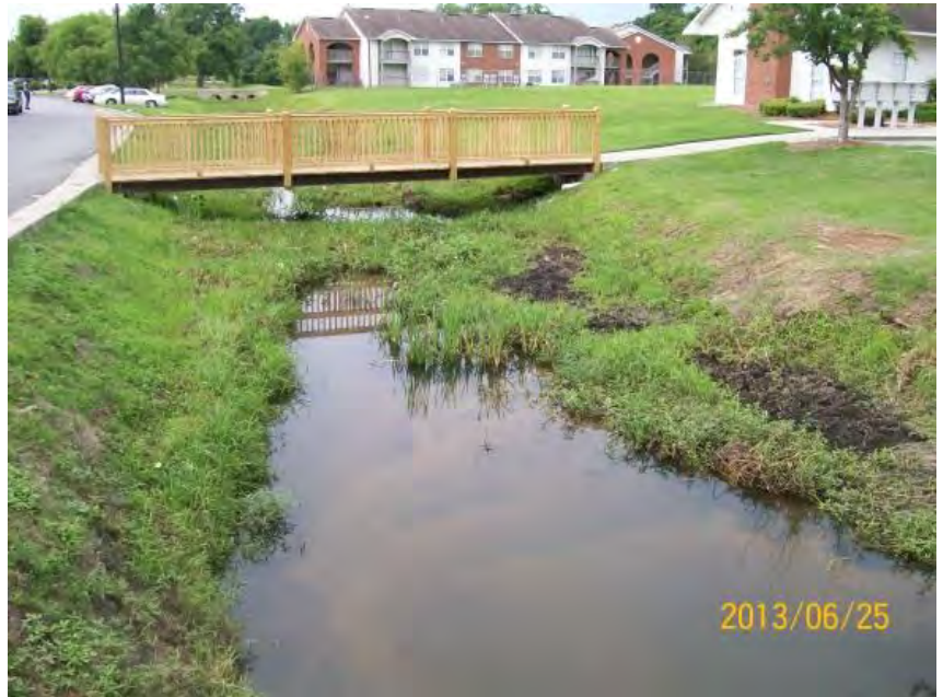
Buildup of silt and vegetation holding water
