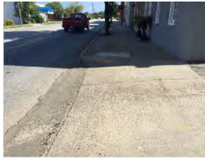
Gutter Filled in at Driveway
