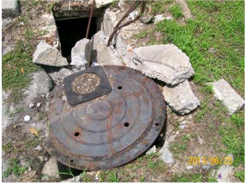
Crushed inlet top
