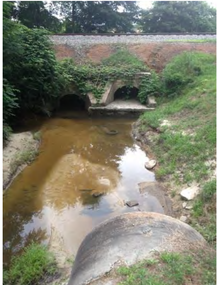
Smaller downstream culverts under rail road
