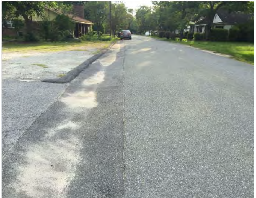
5-feet Wide Asphalt Gutter on South Side of Rountree
