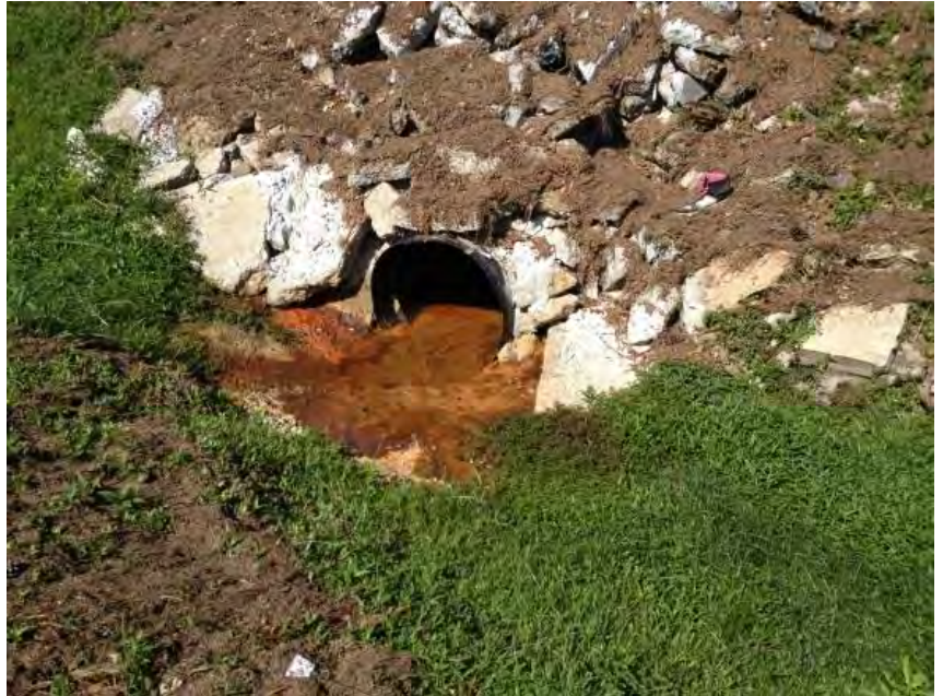
HDPE pipe under Chandler from Ga Villas
