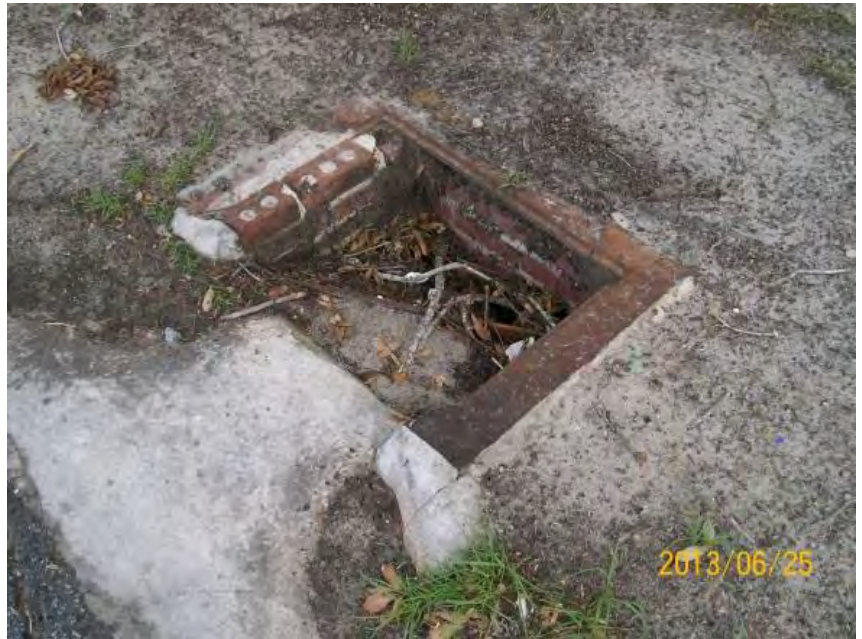
Broken inlet top
