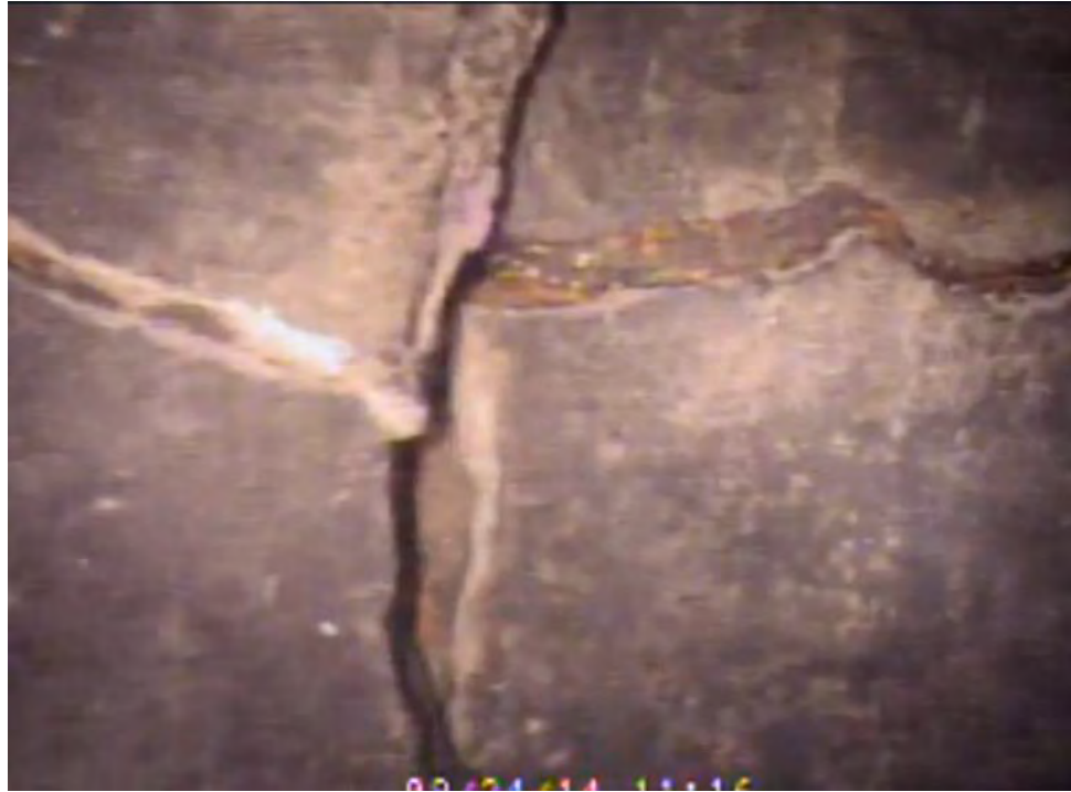
Separation of joint in storm water piping
