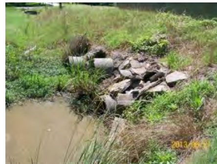
Pipes with no headwall
