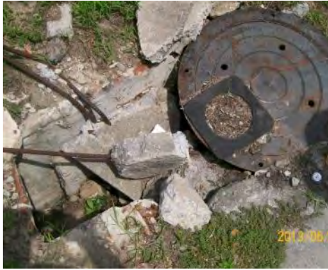
Crushed inlet top
