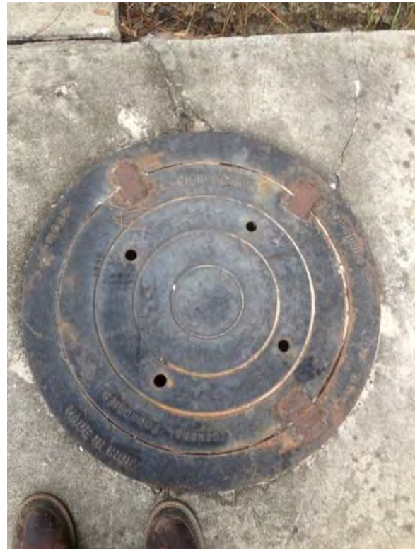
Curb inlet lid welded on
