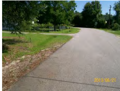
Roadway with shallow swales
