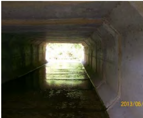
View of box culvert under road
