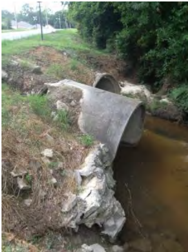
Last section of 84" RCP falling off
