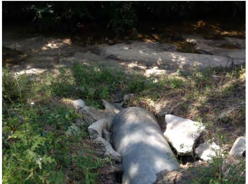
Existing drainage pipe connection from the canal to adjacent low lying area-along the canal.
