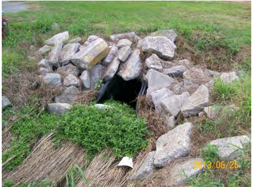
24" HDPE discharge pipe
