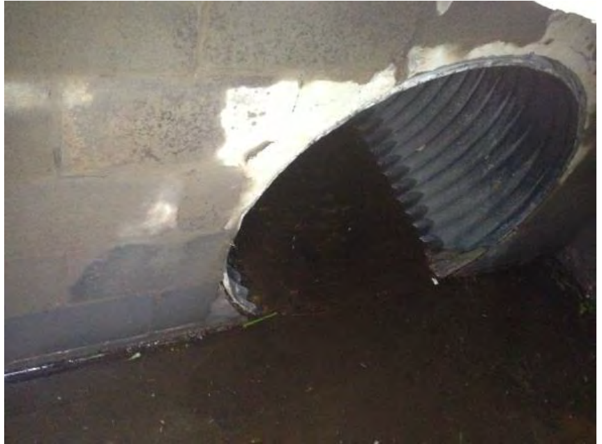
36" CMP constriction in junction box
