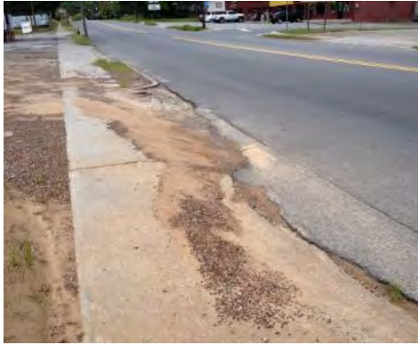
Sediment build up in roadway
