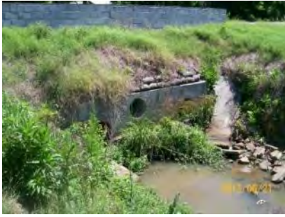
Ditch and pipes with headwall
