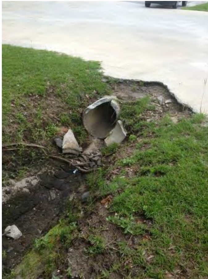
End of pipe broken
