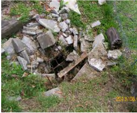
Junction of 15" RCP and 18" HDPE at corner
