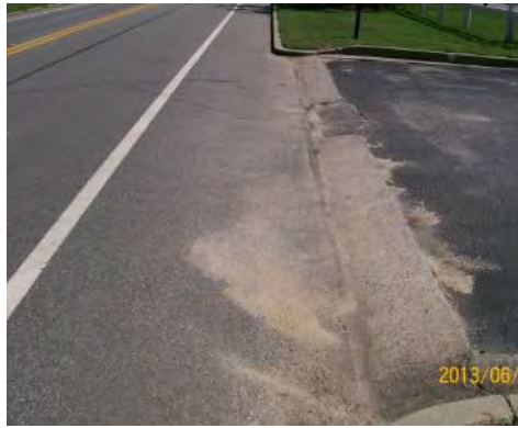
Area where water ponds in gutter.
