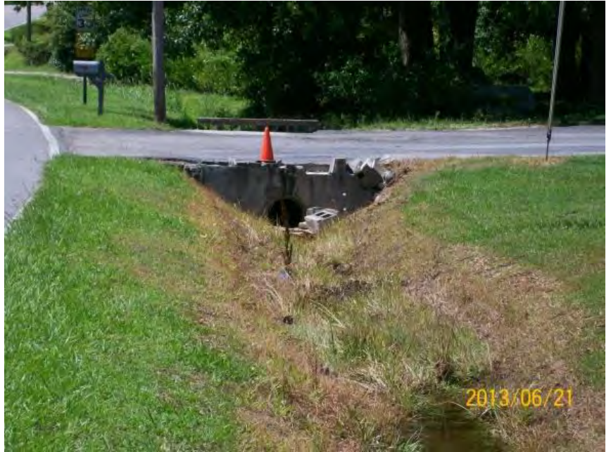
Outfall ditch and downstream pipes
