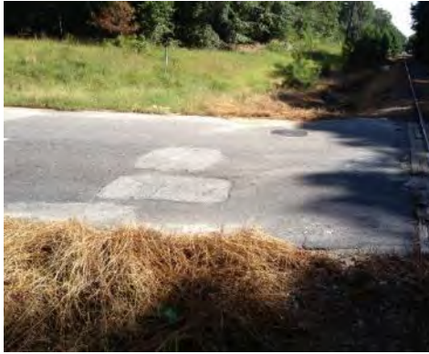
Pavement failing at pipe location
