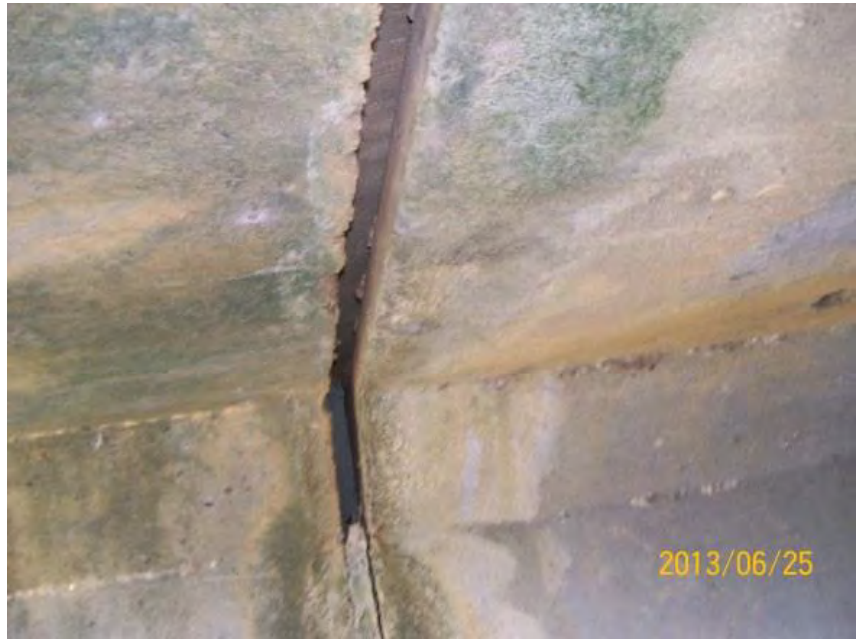
View of leaking joint and missing grout
