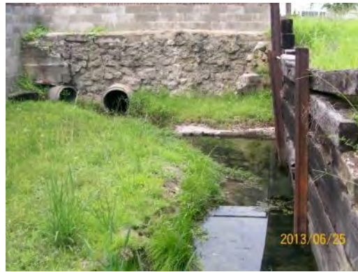
Pipes with headwalls entering ditch
