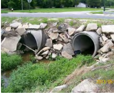
Upstream side in need of headwall
