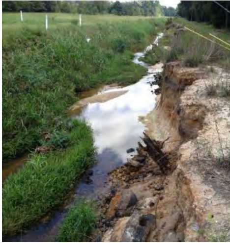
Drainage canal with severe erosion along the bank
