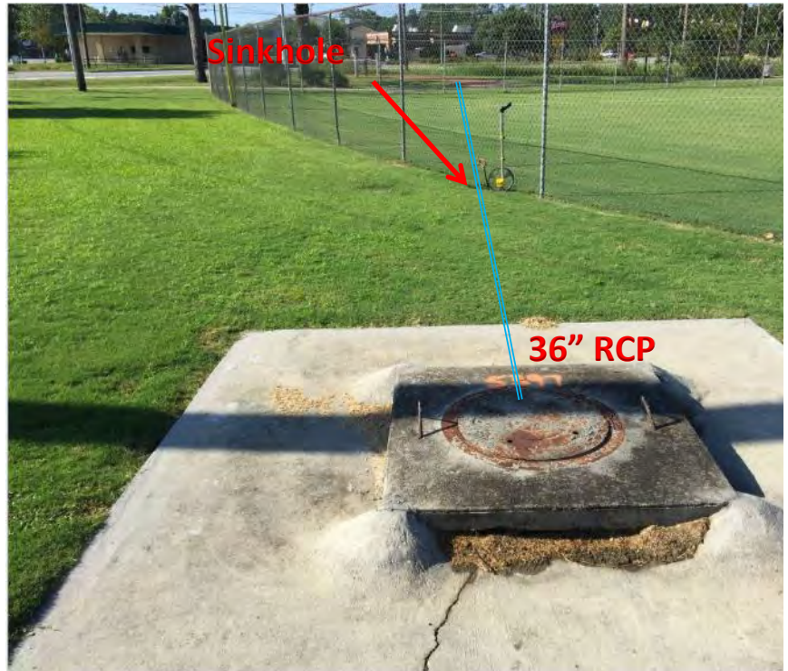
36-inch RCP Under Softball Field, Note Sinkhole
