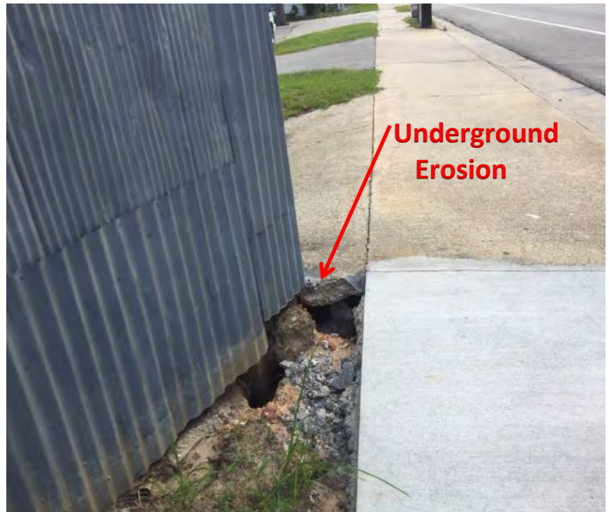
Eroded Hole at Western Corner of Building on Johnson Street
