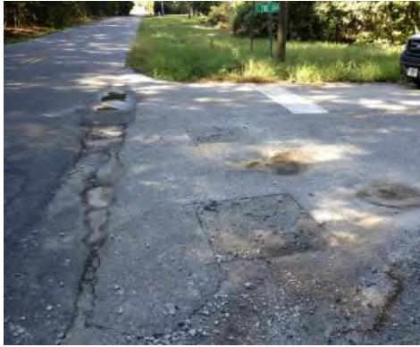
Pavement failing at pipe location
