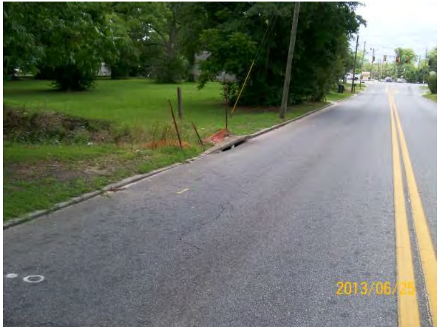
Areas eroded and caving in around catch basin
