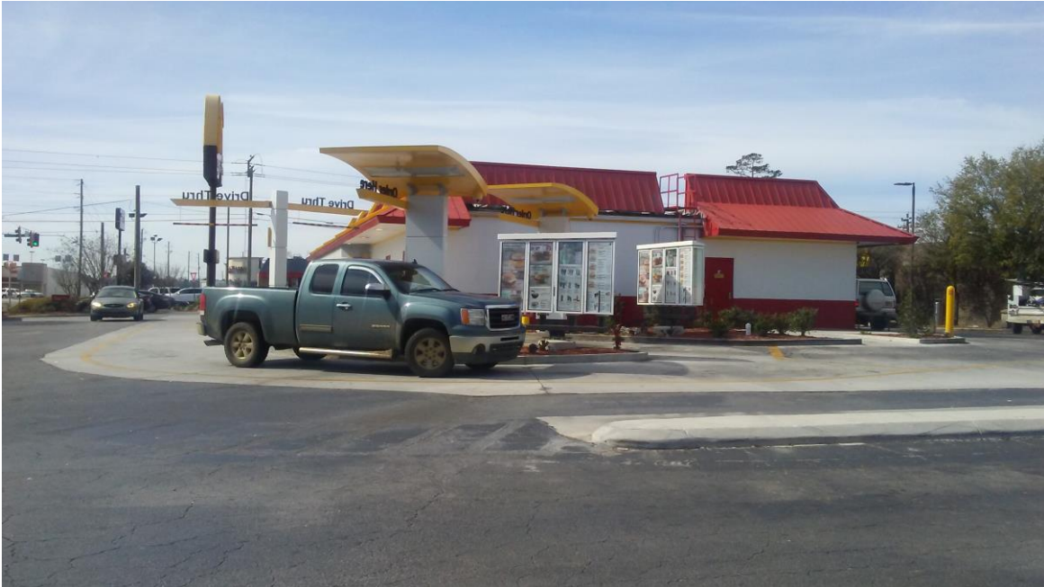
Picture 5 Rear of Subject Site Depicting Menu Boards
