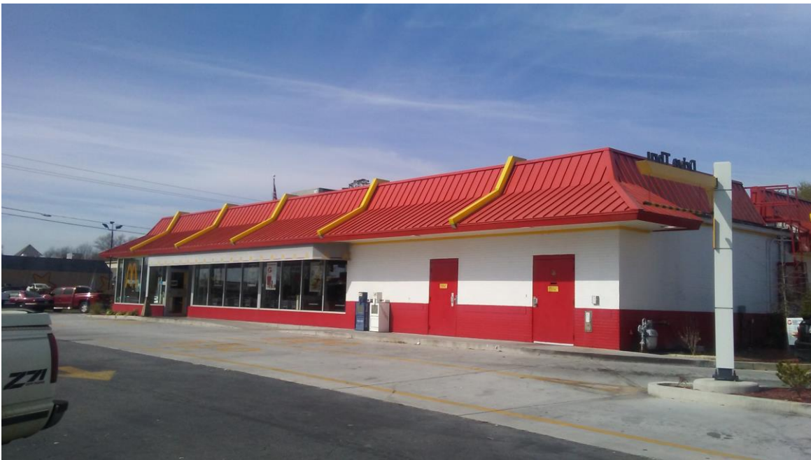
Picture 2 Subject Site Non-Drive-thru Side facing Parking Lot and Lovett Road
