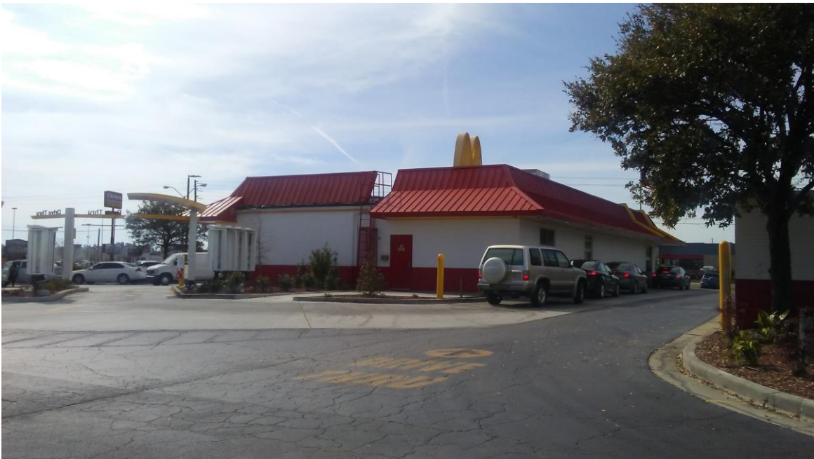
Picture 6 Rear Elevation of Subject Site
