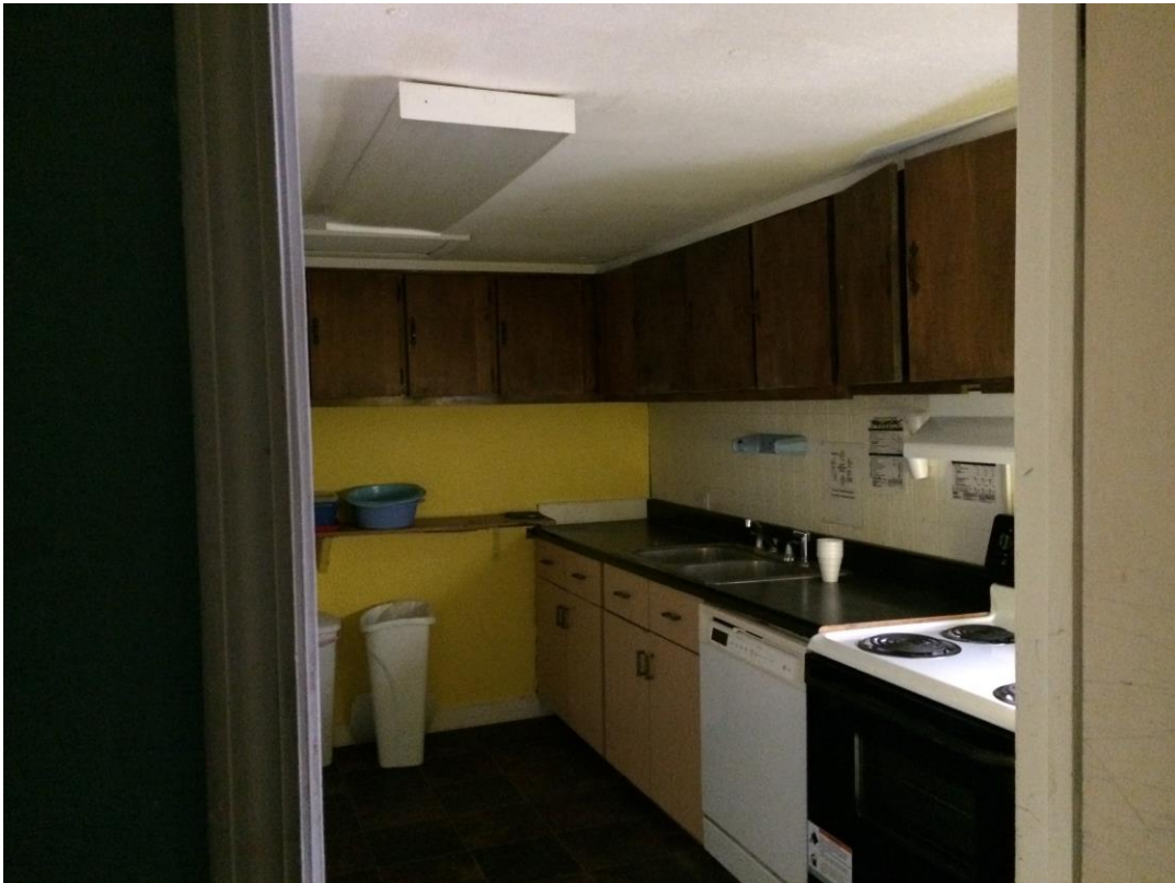
Picture 14 Interior of Subject Site Depicting Kitchen Area
