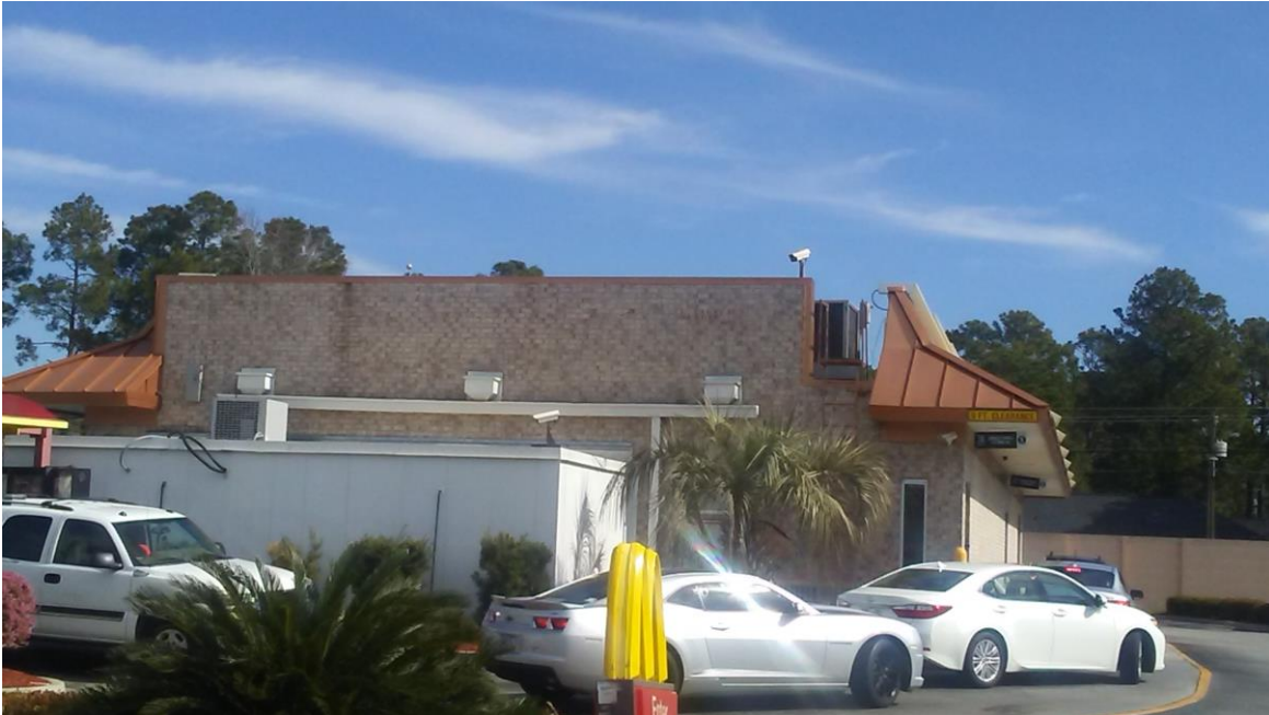
Picture 3 Rear Elevation and Directional Signage
