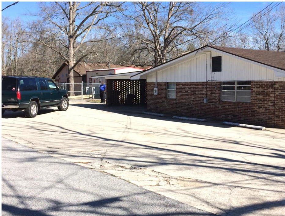
Picture 4 707 West Jones Avenue facing North East Depicting Portion of the Parking Lot
