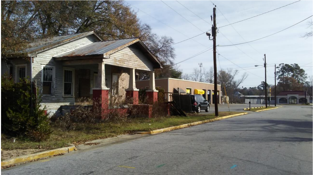
Picture 9 Single-Family Dwelling and Meineke Car Care Center facing east toward South Main Street
