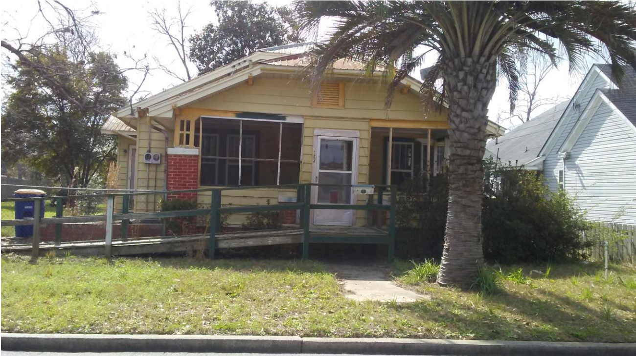
Picture 1: Subject Site from West Inman Street facing South
