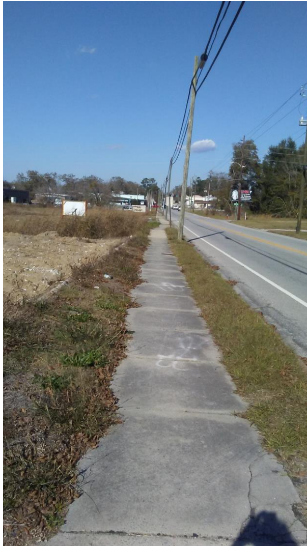
Picture 2: Subject Site Depicting South College Street and Existing Sidewalk facing North
