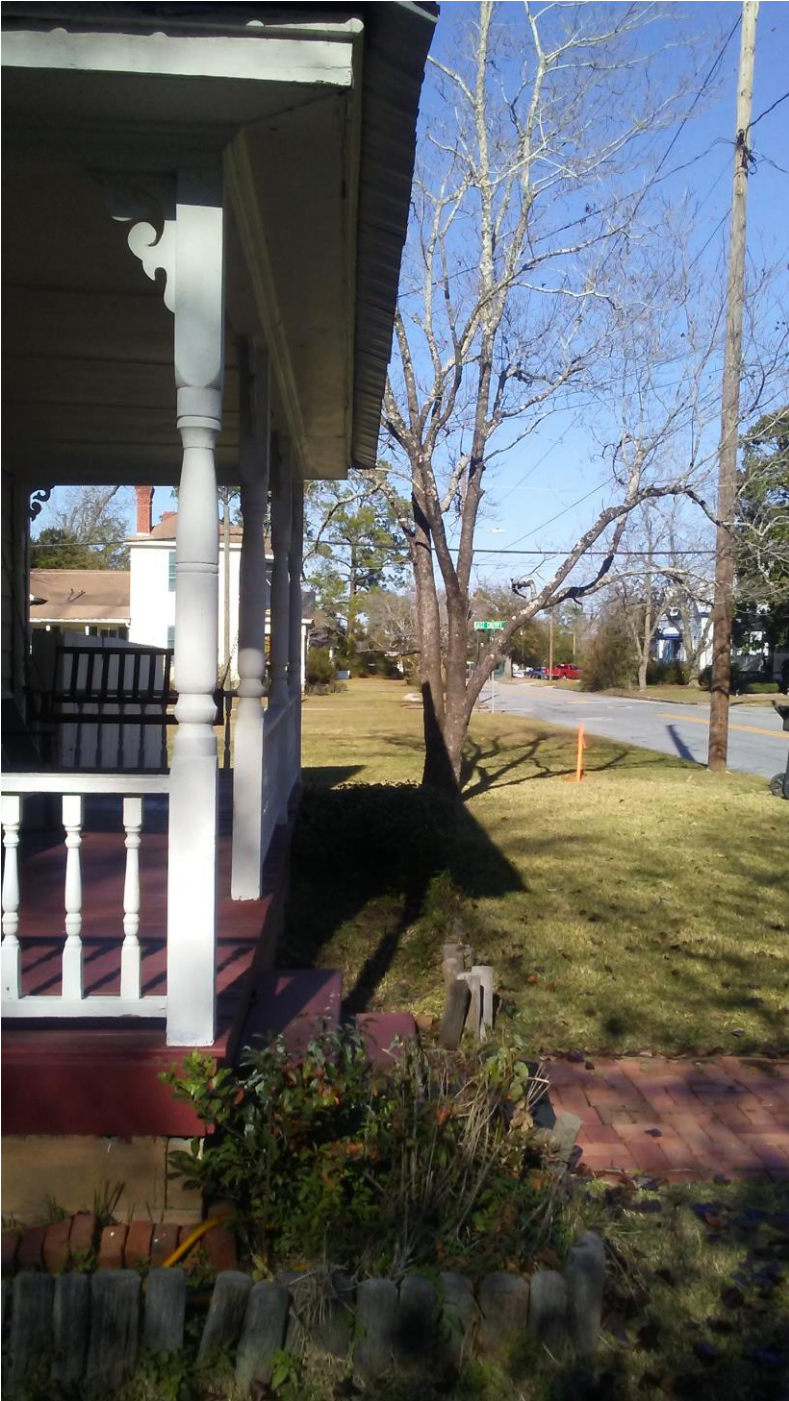
Picture 6: Porch of Single-Family Dwelling at 105 Broad Street Depicting Setback
