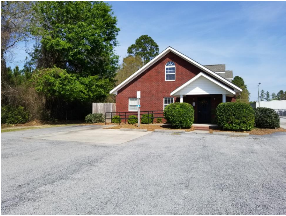
Picture 6: Rear Elevation of Subject Site
