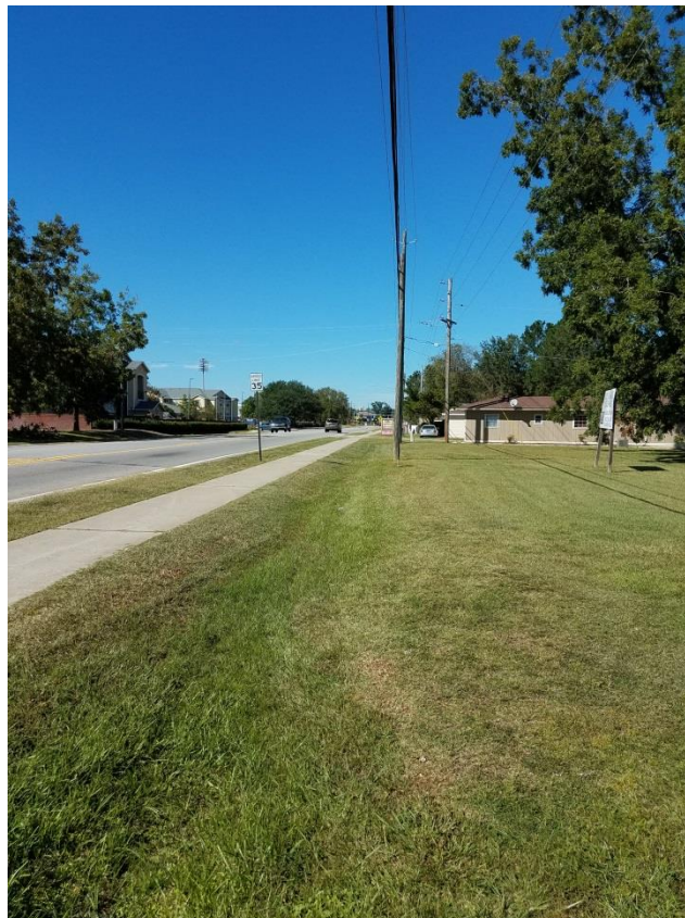
Figure 6: Subject Site Facing North Depicting Lanier Drive
