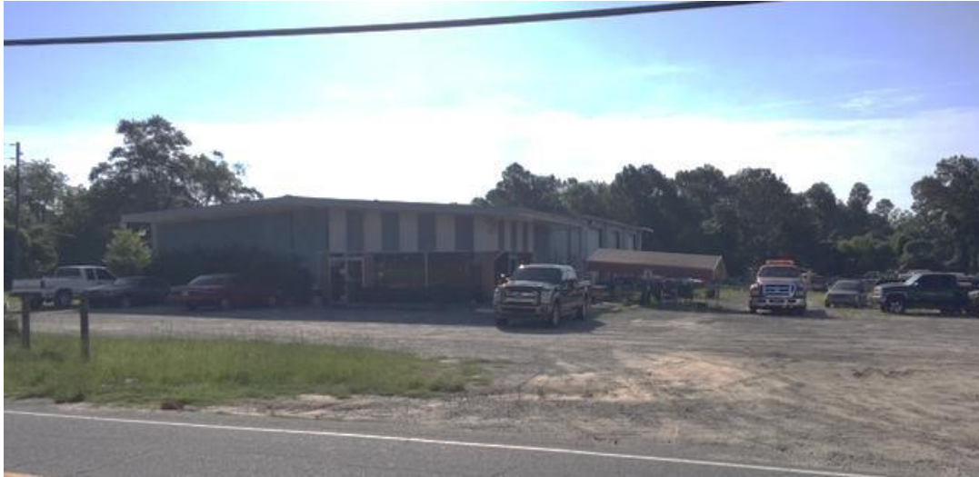
Picture 2: Looking south, a portion of the subject site & adjacent structure to the south, currently a church
