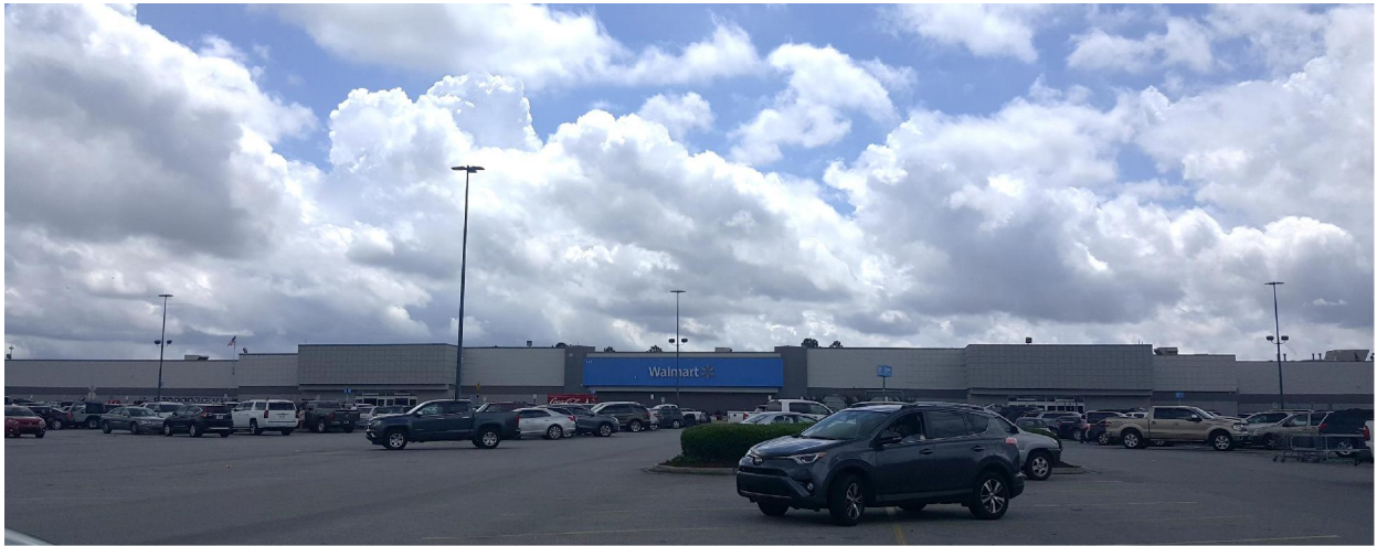
Picture2: Subject Site depicting proposed location for additional signage (orange section), right side of front elevation.
