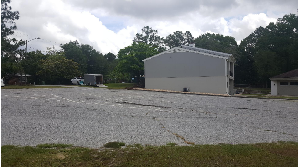
Picture 1: Subject Site from Fair Road facing east, showing the proposed signage location
