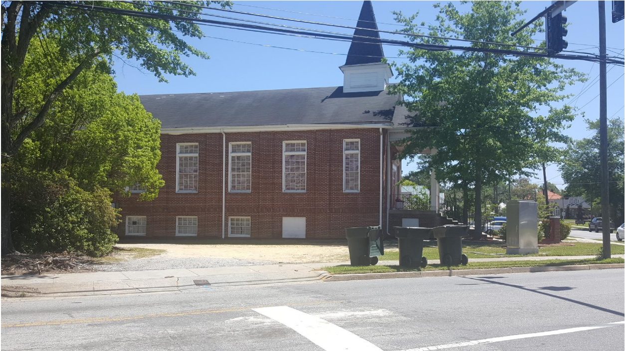
Picture 4: Subject site depicting side elevation along Zetterower Ave facing east
