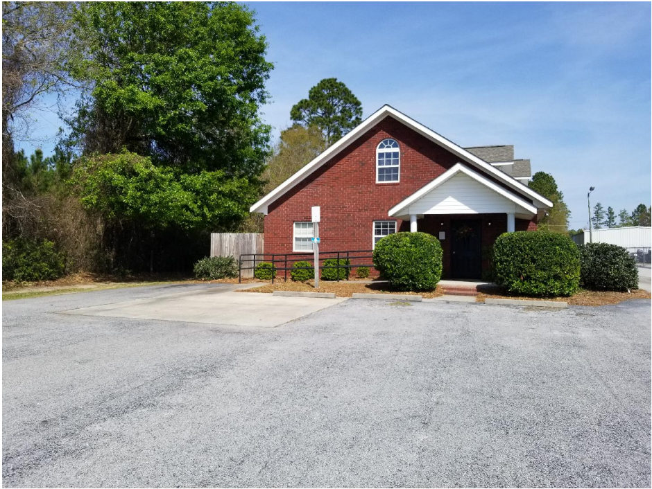
Picture 6: Rear Elevation of Subject Site
