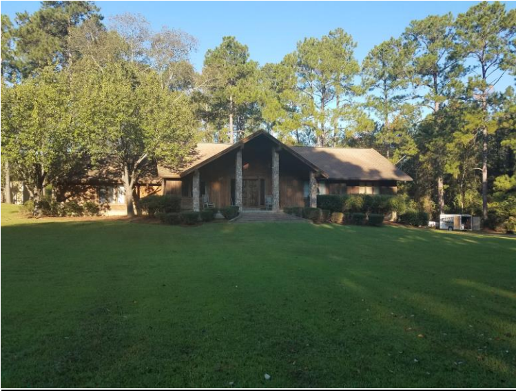
Picture 1 Front Elevation of Subject Site Facing West
