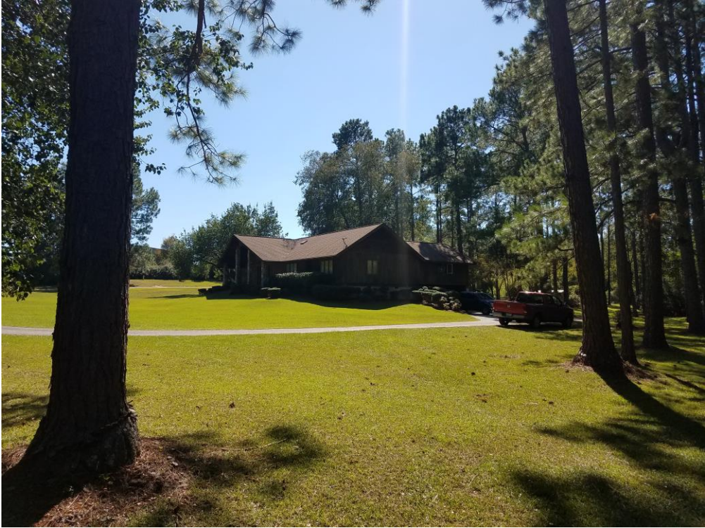
Picture 2 Side Elevation of Subject Site Facing Southeast
