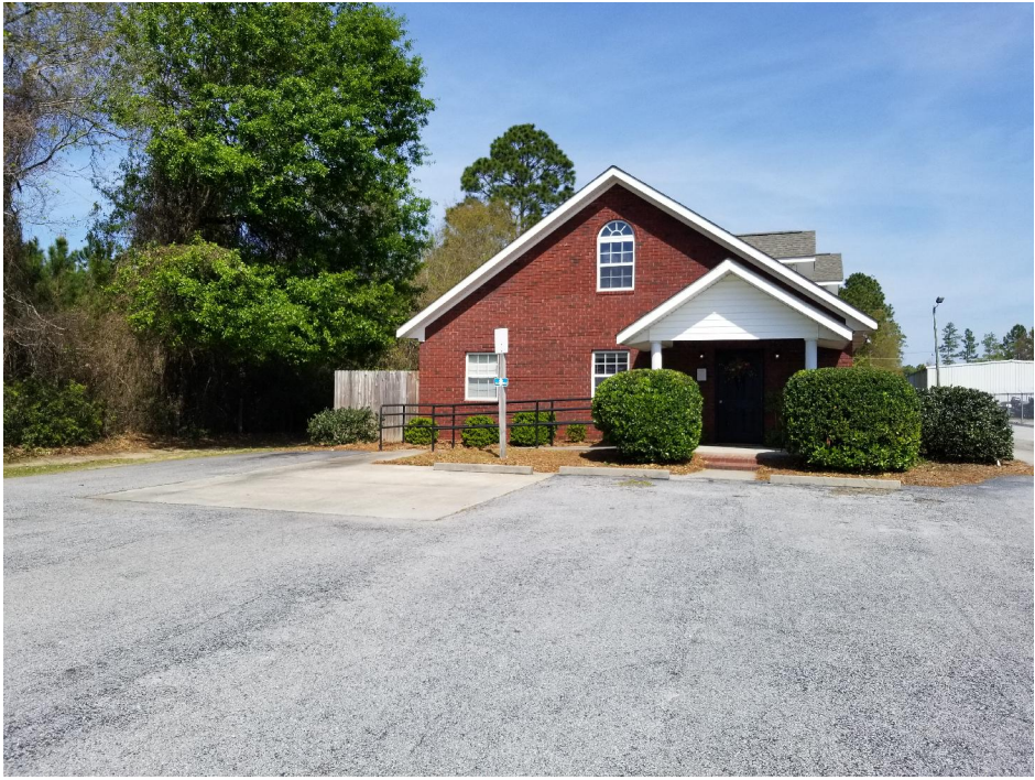
Picture 6: Rear Elevation of Subject Site
