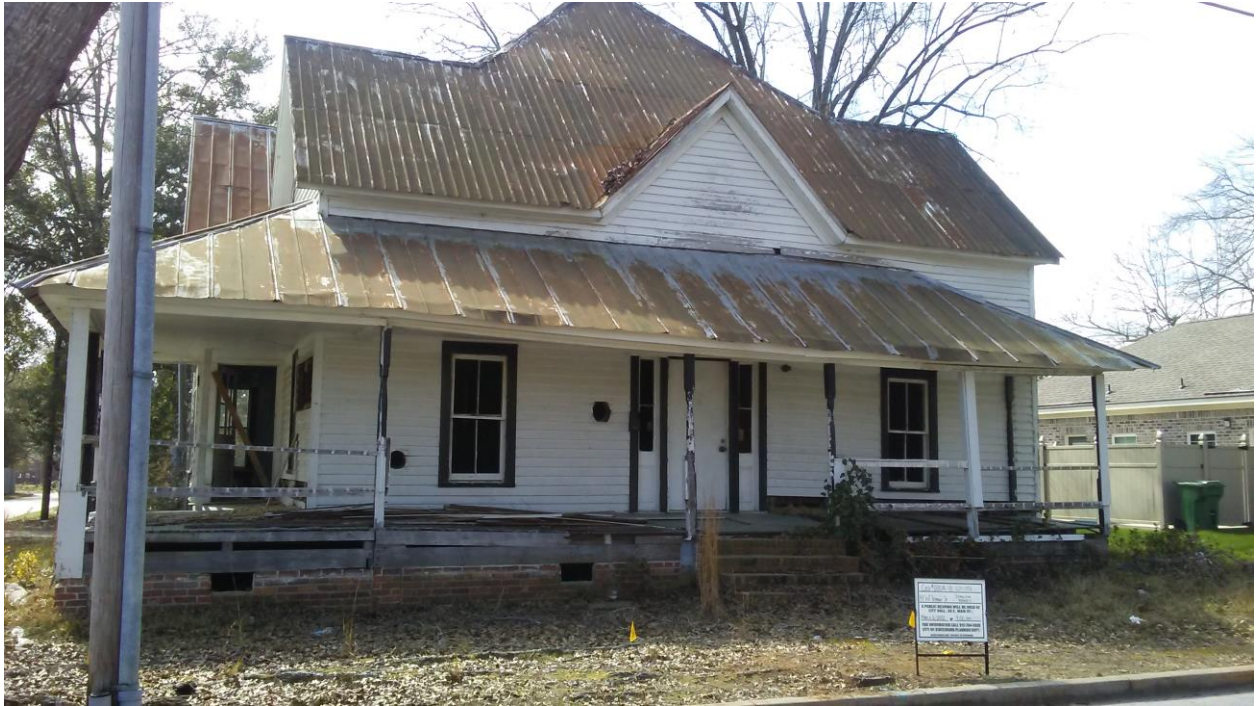
Picture 2: Subject site depicting front elevation along West Inman Street facing South
