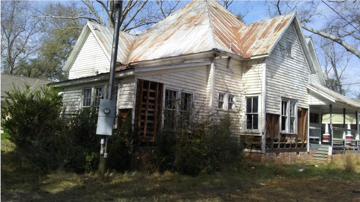
Picture 4: Subject site depicting rear and side elevations
