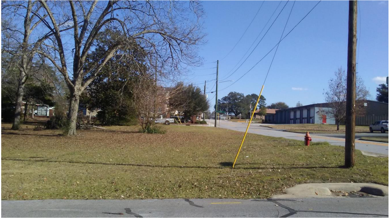
Picture 2: Subject Site from Institute Lane Facing East
