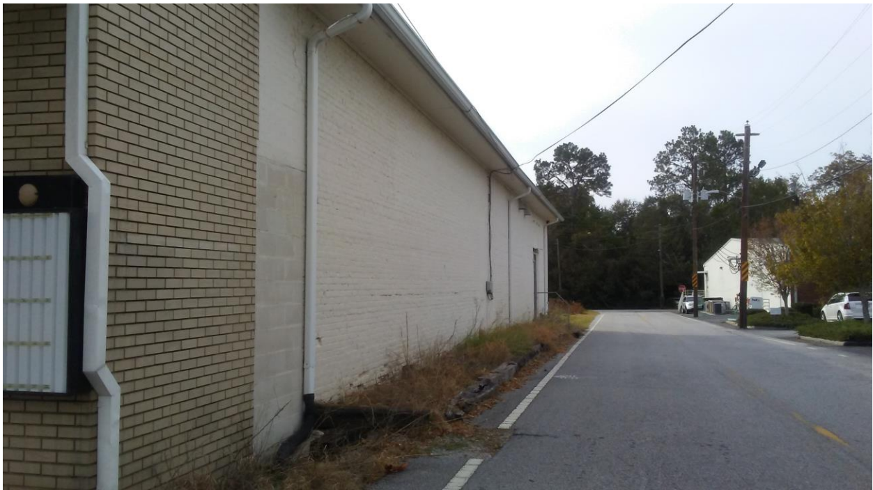
Picture 4 West Exterior Wall Depicting Proposed Alley Closure Connecting Cherry Street and East Vine Street
