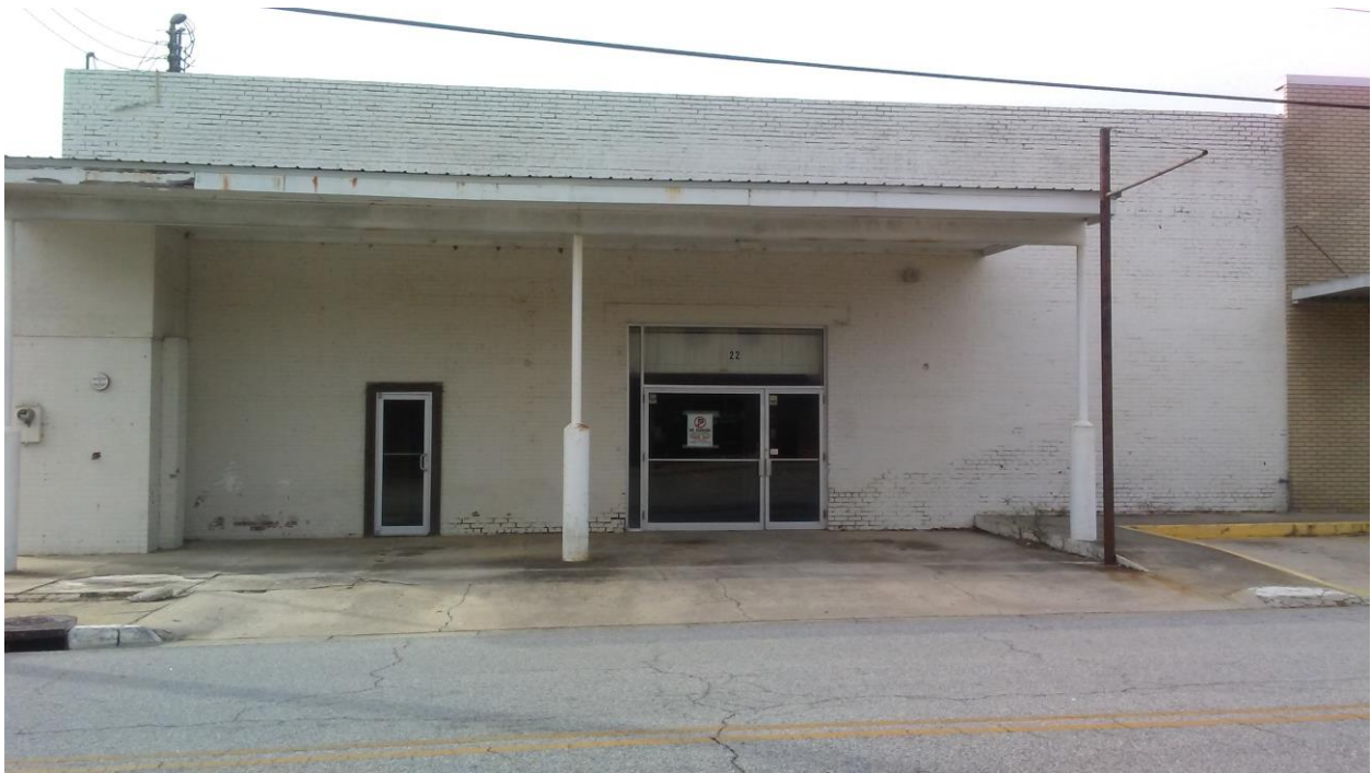
Picture 2 Exterior of 22 East Vine Street
