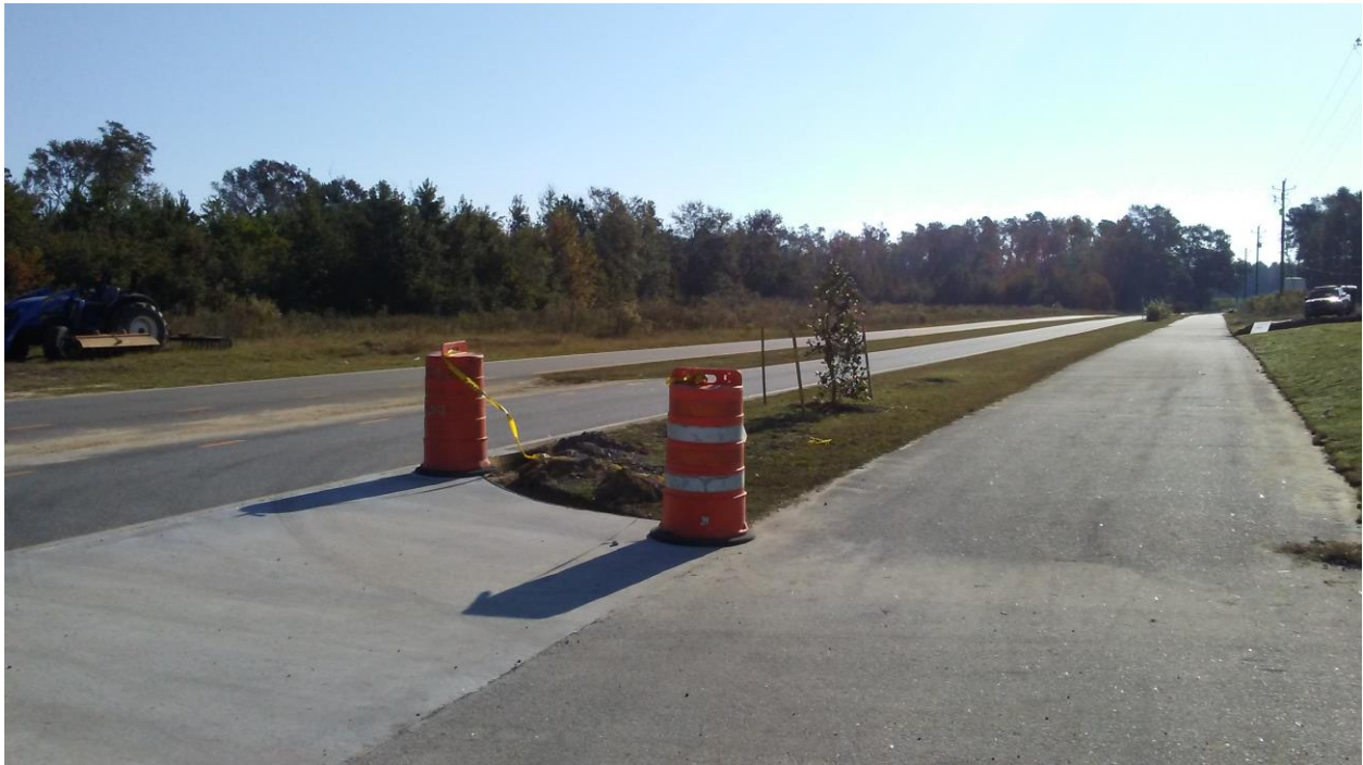
Picture 4 S & S Railroad Bed Road Facing South East at Entrance of Development
