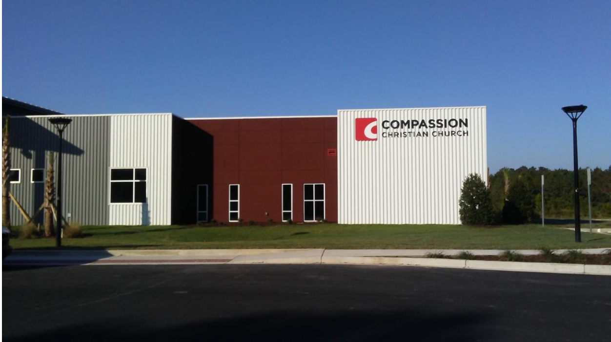
Picture 1 Installed Building Sign at 73.35 Square Feet
