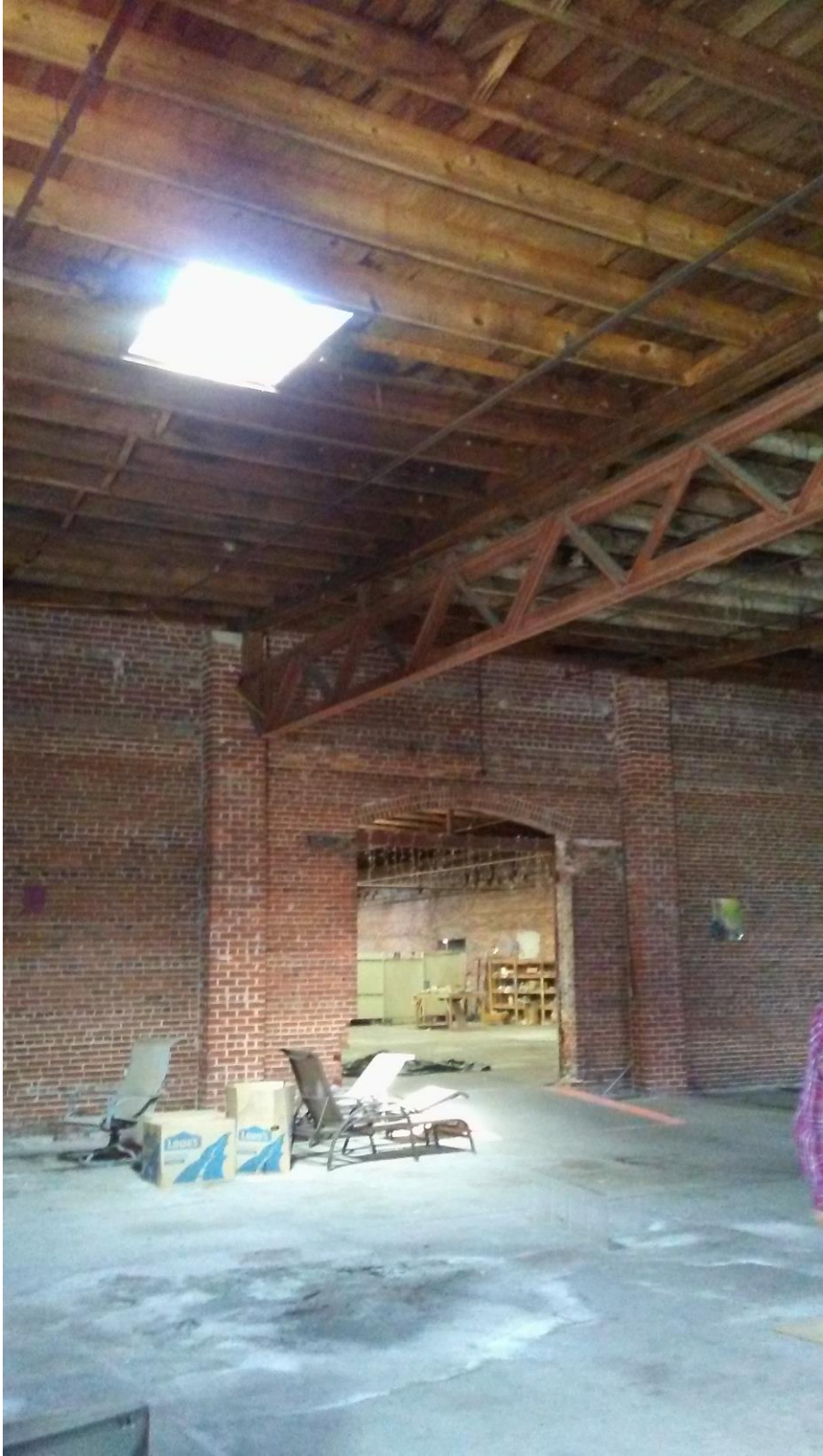
Picture 9 Interior Depicting Archway, Skylight, Masonry and Exposed Beams
