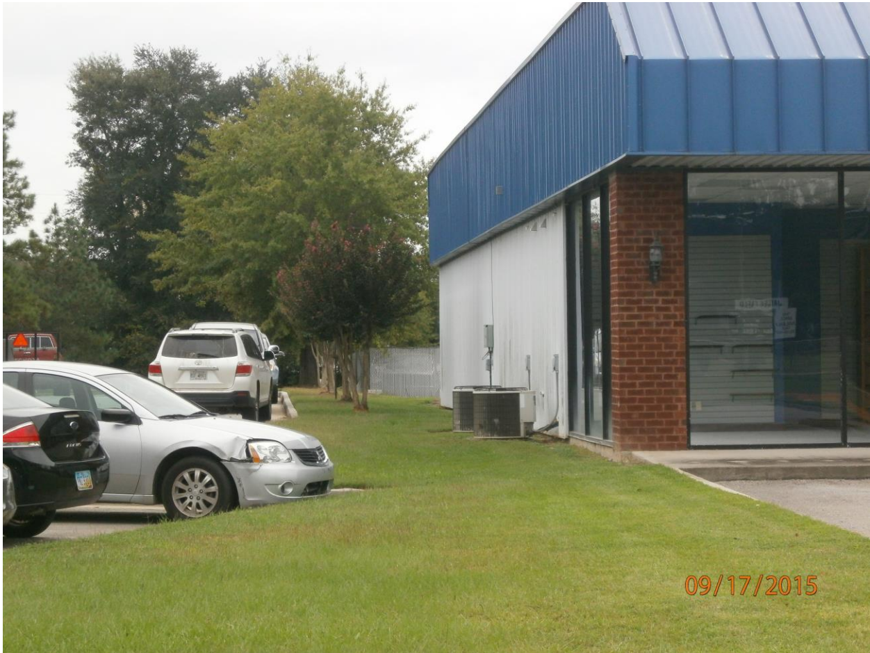
North edge of building along existing 5' setback limit.
