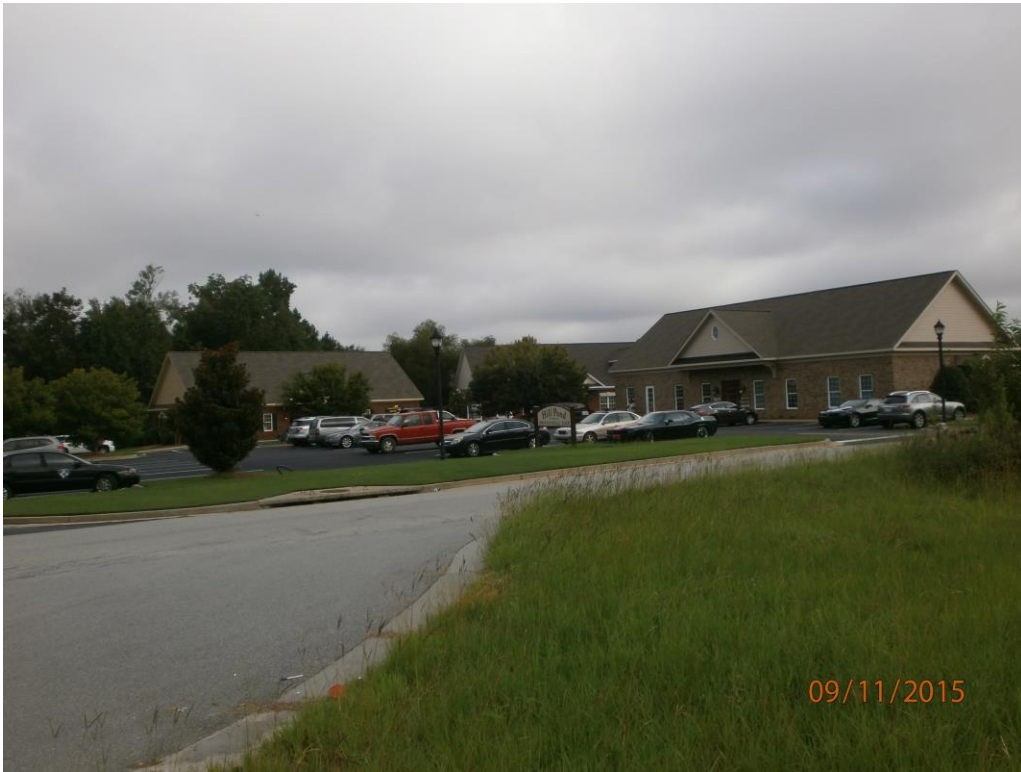
Picture 10 Northern Portion (CR) of Subject Site Facing Hill Pond Professional Park
