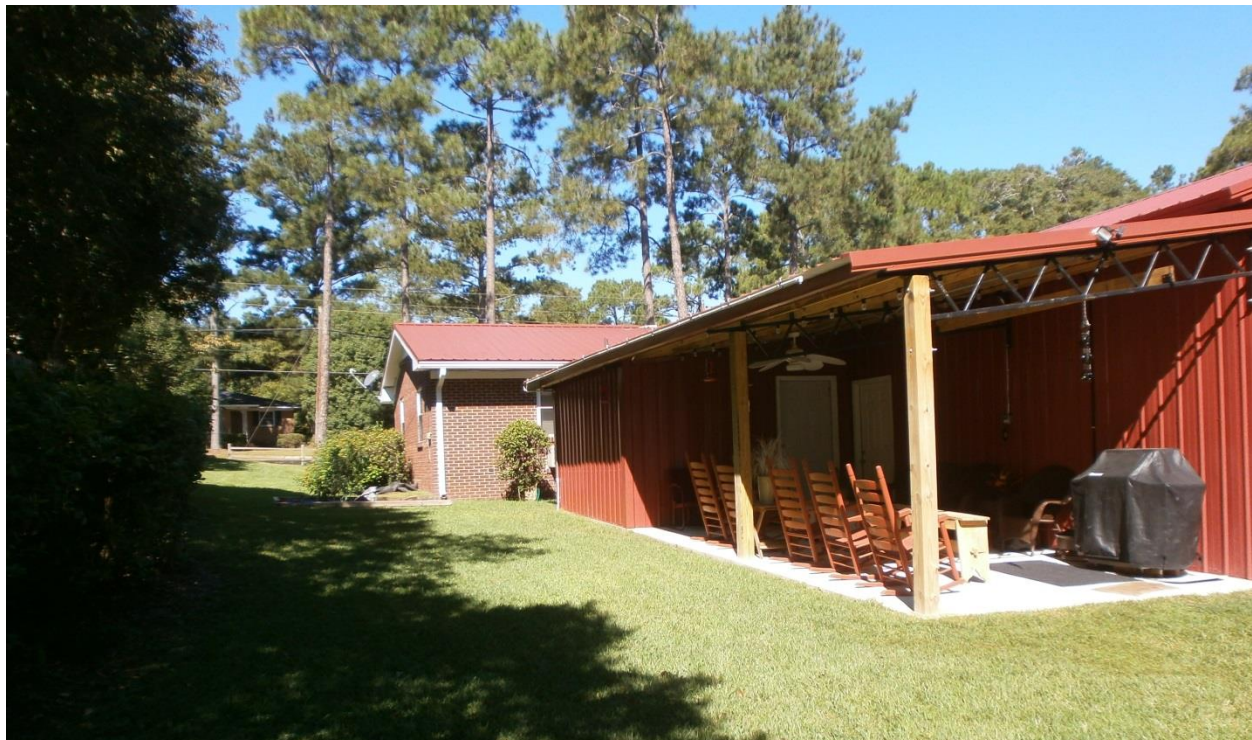
PHOTO 6: South Side Yard View from the Inner Corner of the Rear Yard of Subject Site. Wooden Privacy Fence is to the left behind the shrub bushes. Porch is the back side of the Attached Carport
