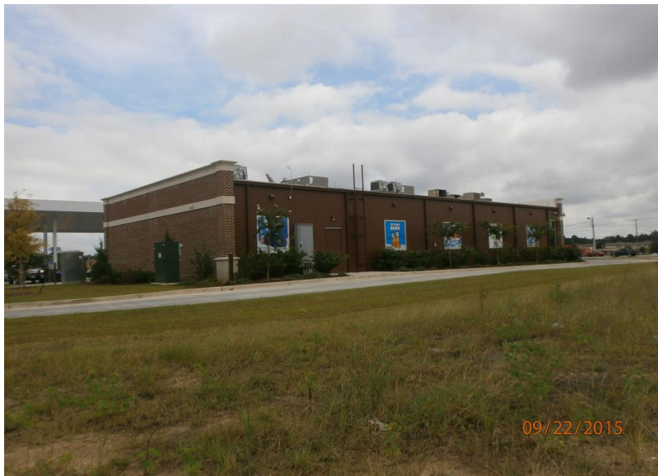
Picture 6 Parker's Located on Lot 1 of the Subject Property Facing West
