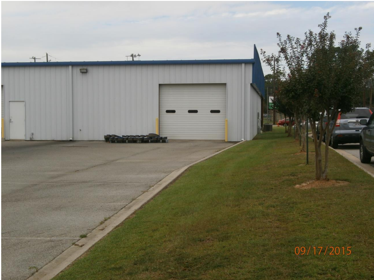
Rear view of building along 5' setback limit.
