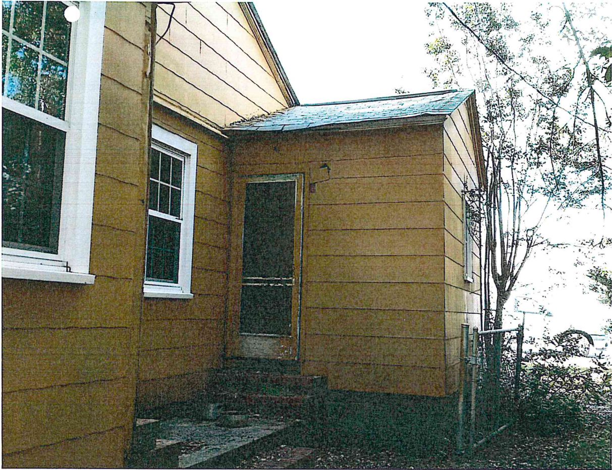
Picture 5 Rear of Subject Site
