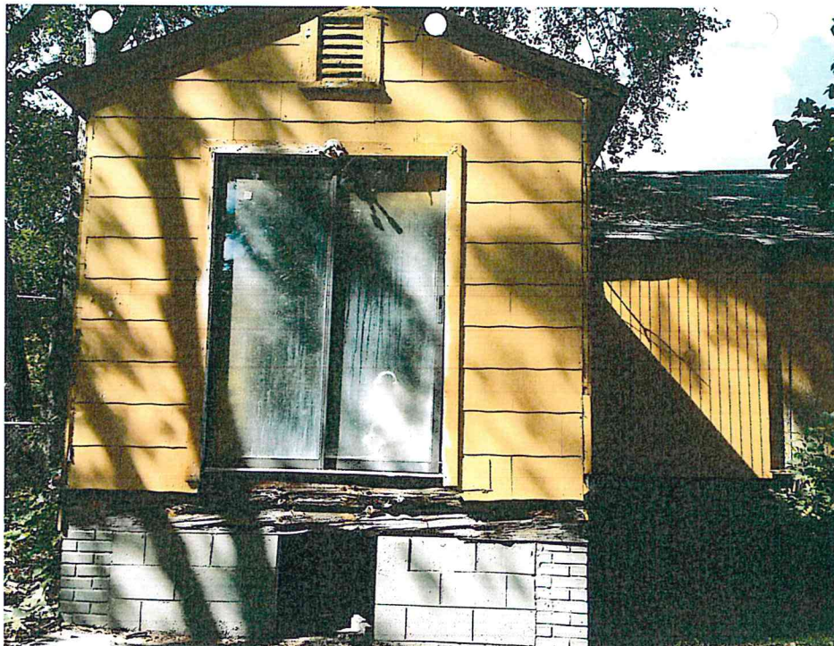
Picture 7 Rear of Subject Site
