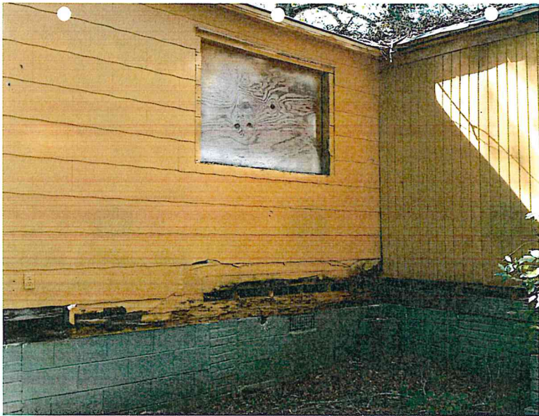
Picture 6 Rear of Subject Site
