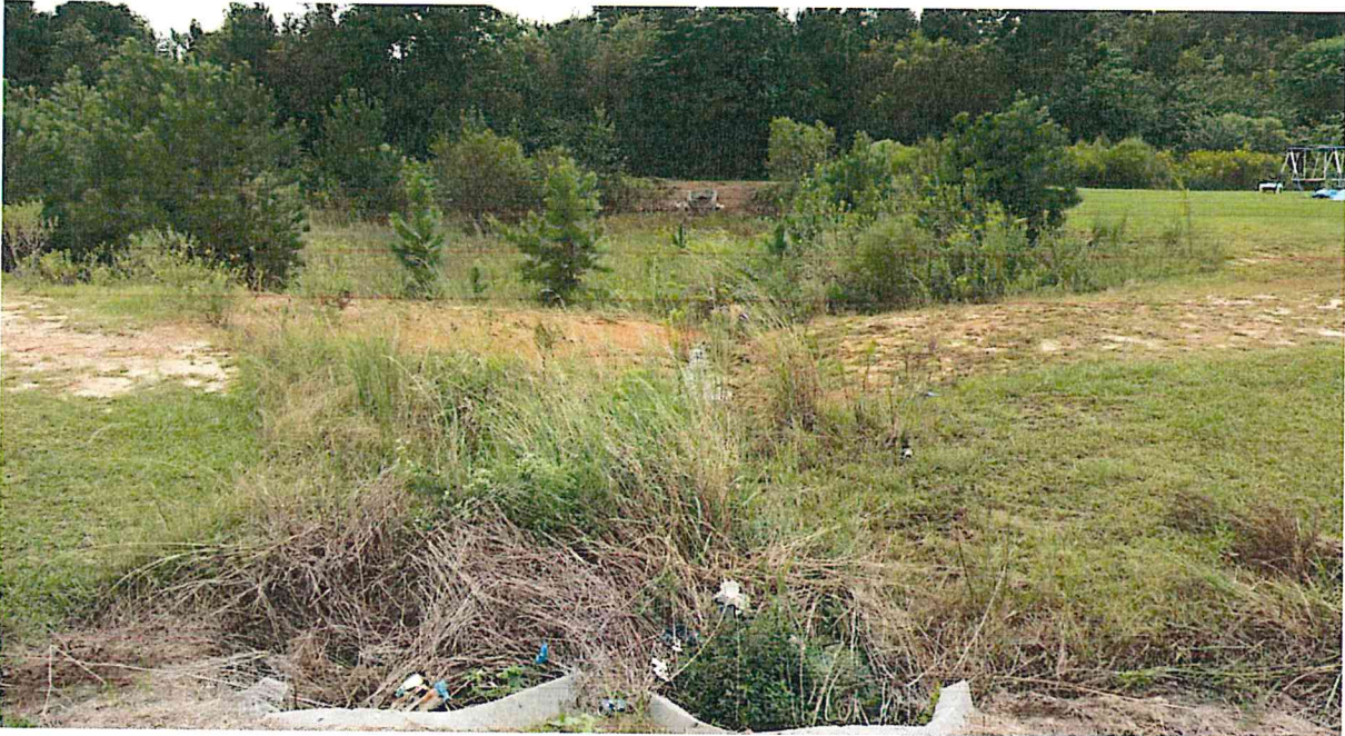
Detention Pond between Existing Lots 5 & 6
