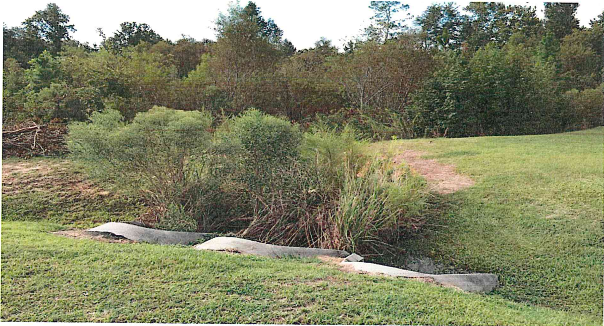
Detention Pond & Drainage located on Scotch Pine Ave between Lots 22 & 23
