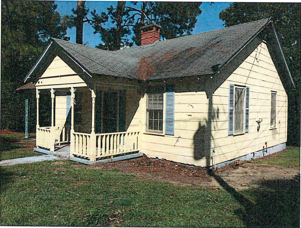
Picture 2 Front of House Facing South
