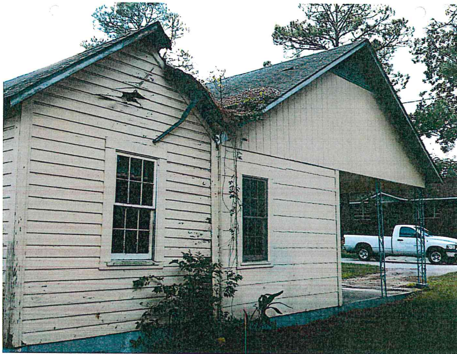
Picture 4 Rear of Subject Site
