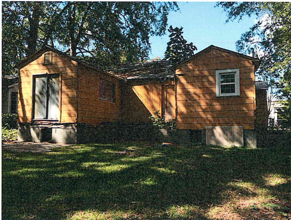
Picture 4 Rear of Subject Site
