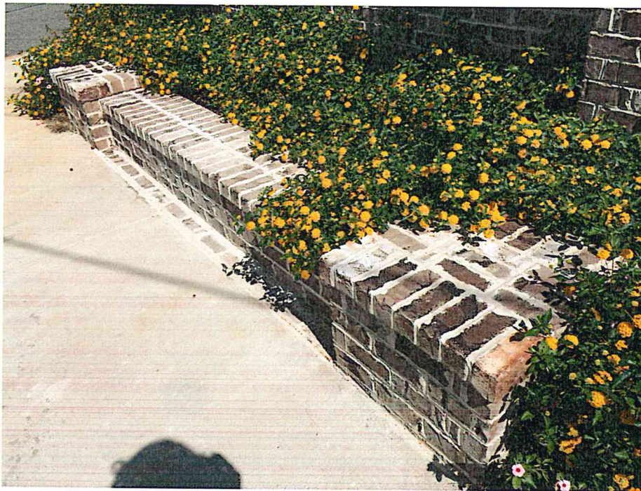
Picture 4 Installation 8" up to Property Line on Left Side of Sign (Upper Corner of Picture)
