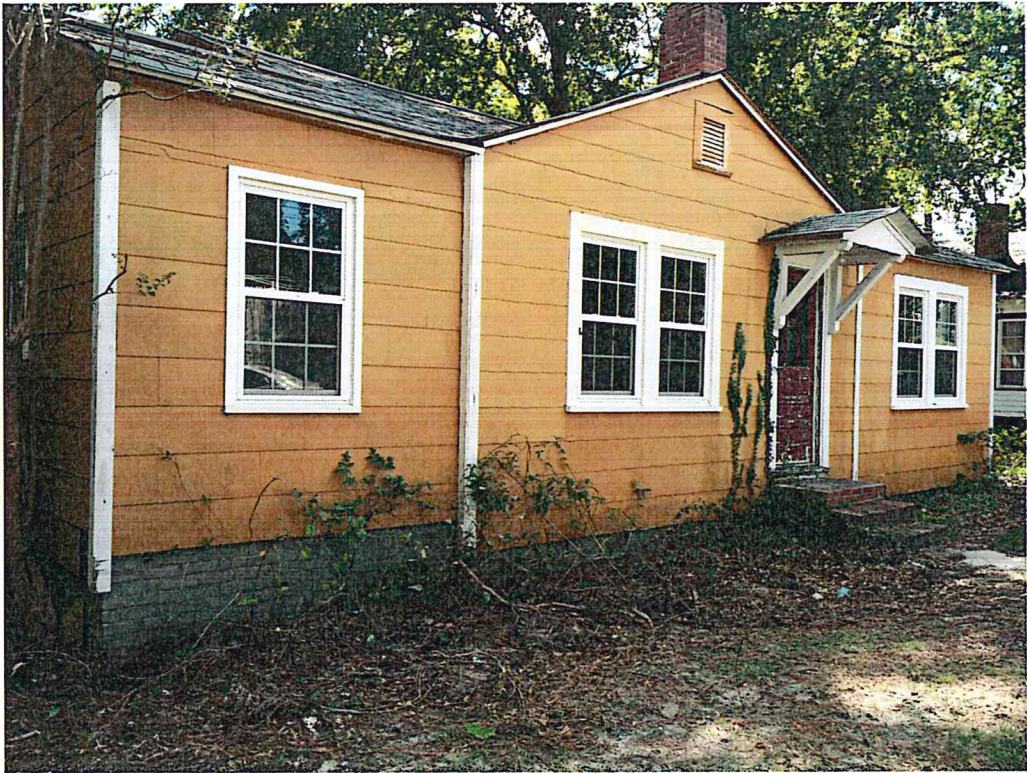
Picture 2 Front of House Facing South
