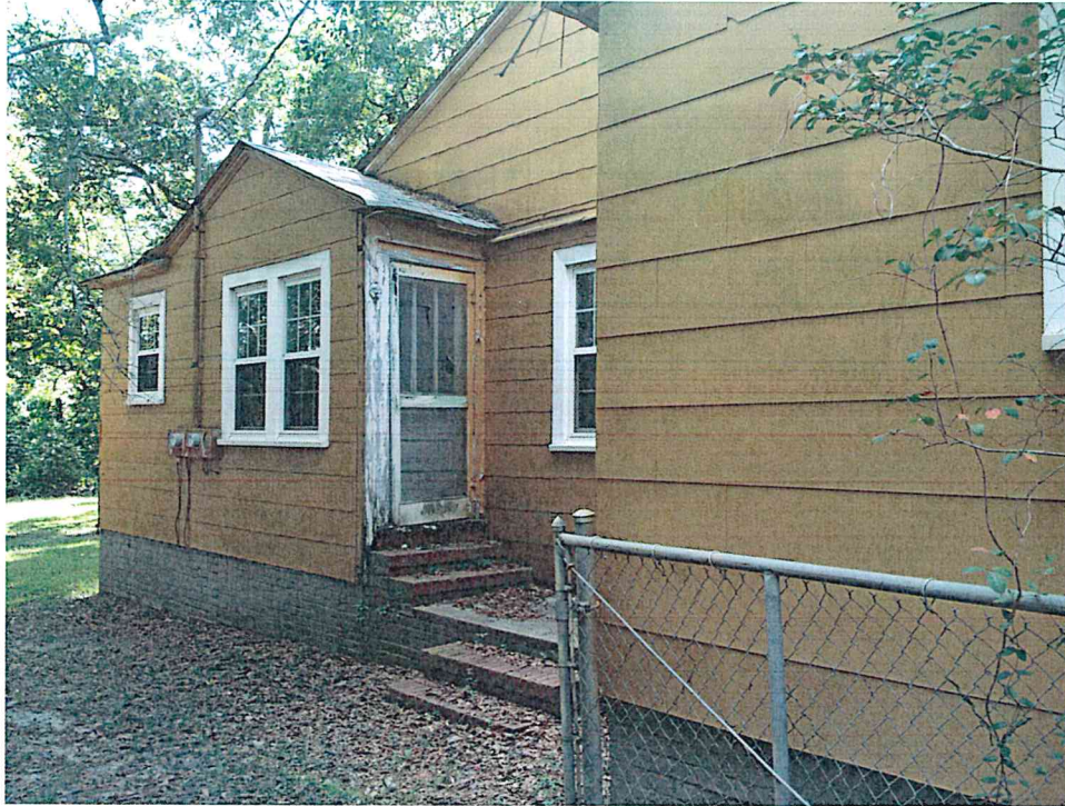
Picture 3 Rear of Subject Site
