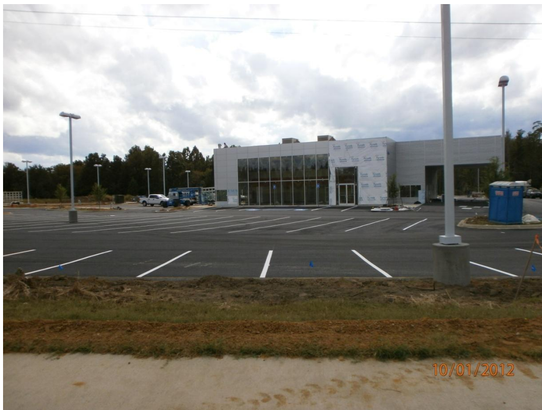
Figure 2: The Subject Property under Construction from Brannen Street.
