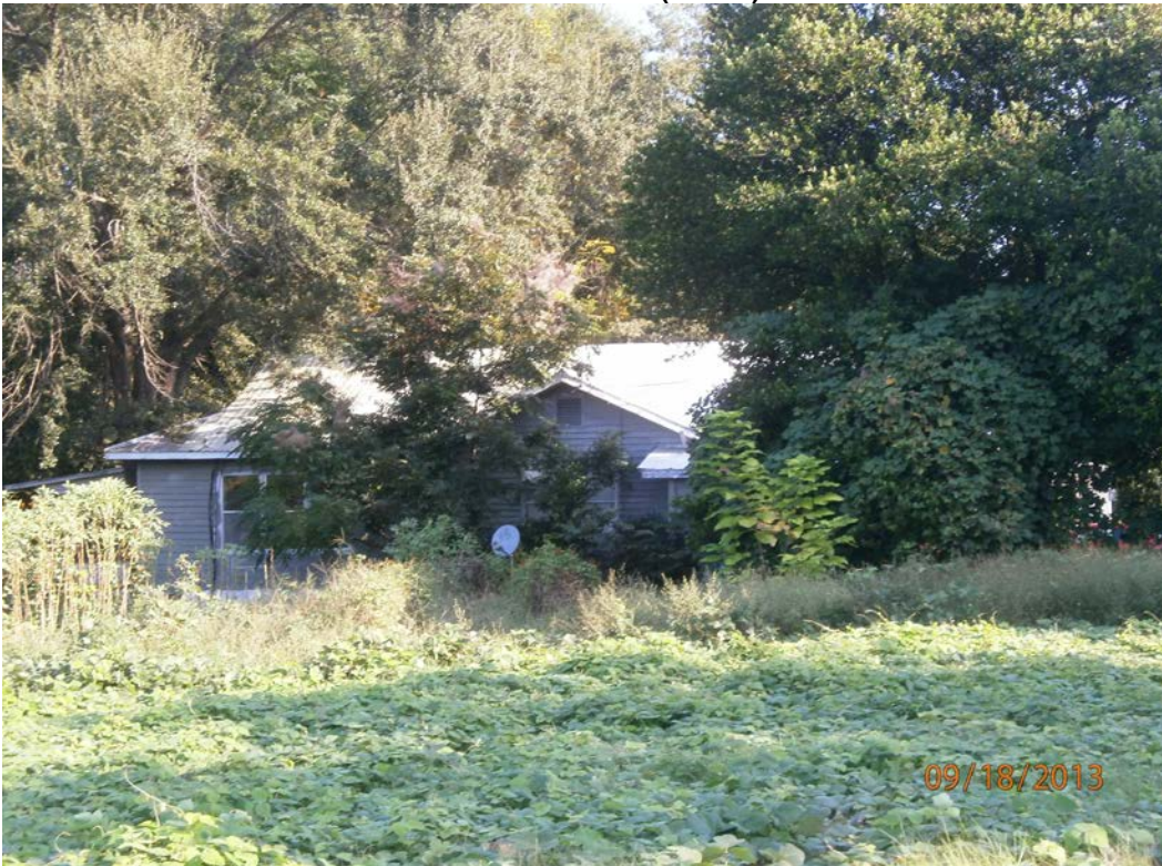
Figure 3: Northern view, connects to single family residence.
