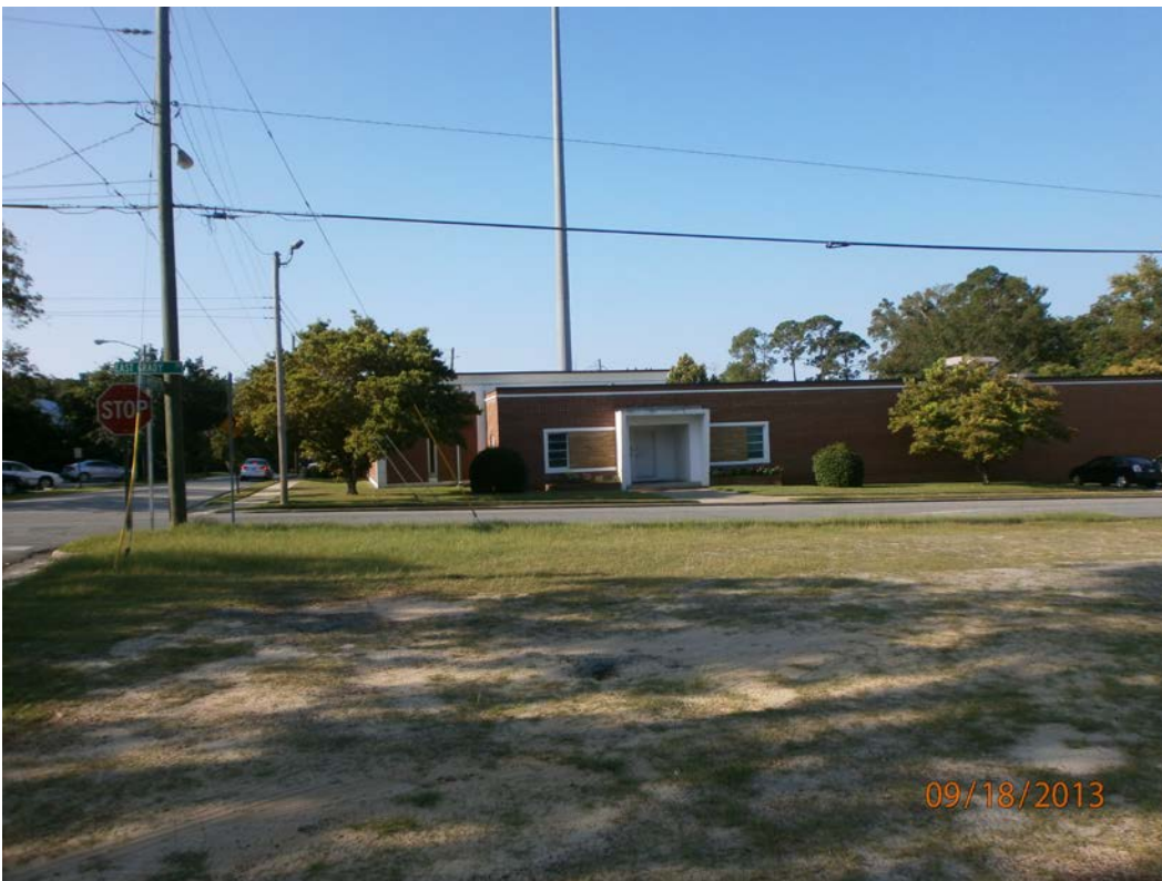
Figure 4: Southern view, fronts E. Grady Street, facing FRONTIER COMMUNICATIONS.
