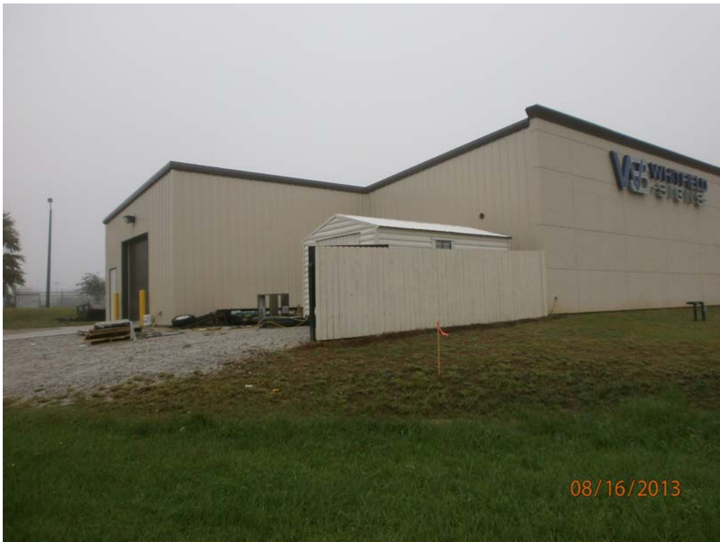
Figure 2: Subject Site rear northwestern view.
