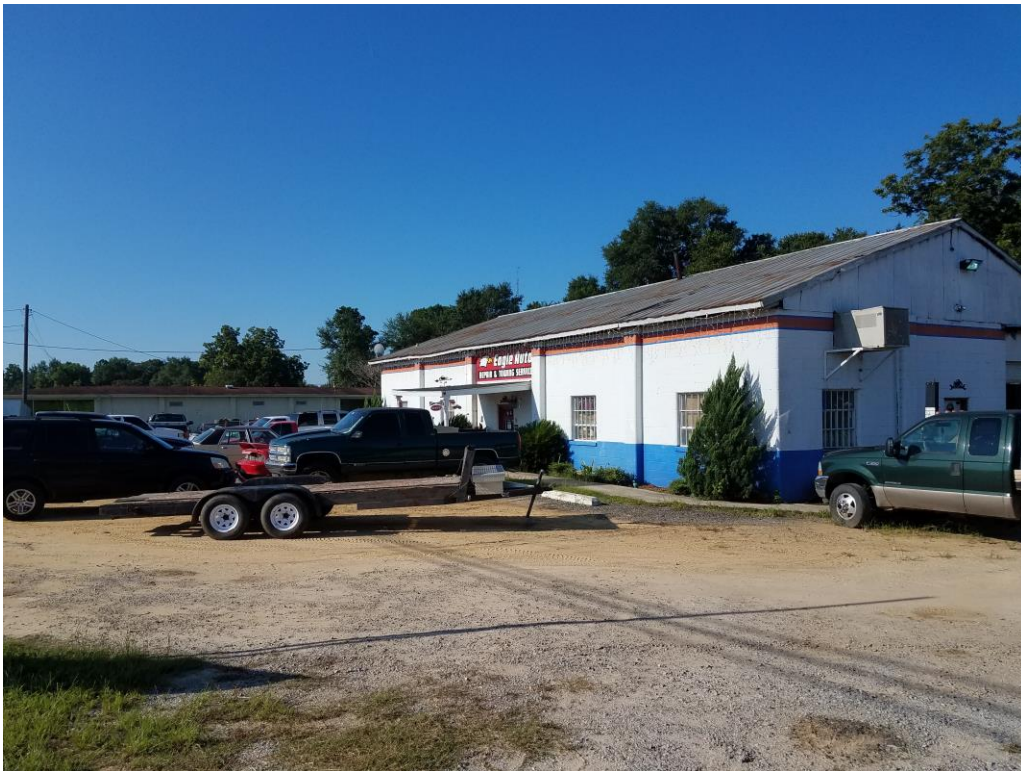
Picture 2 Subject Property Facing South
