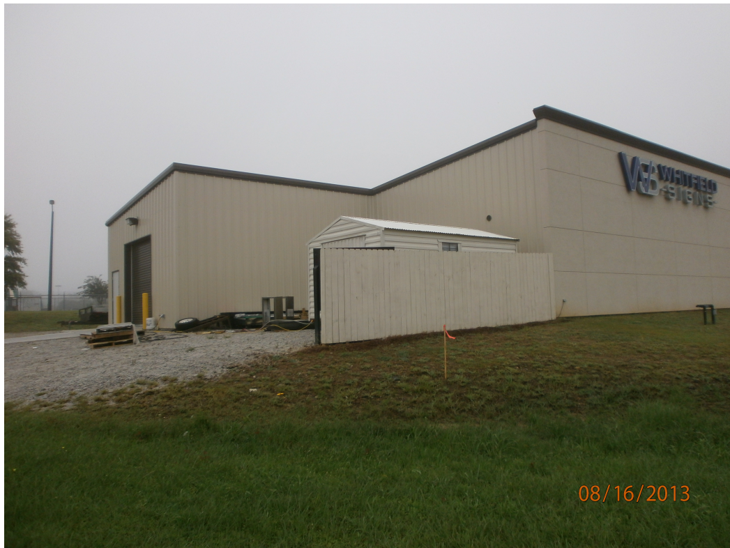
Figure 2: Subject Site rear northwestern view.
