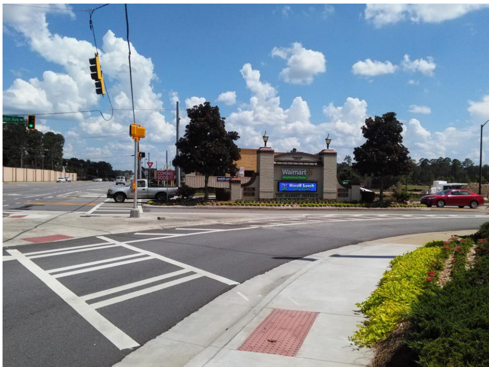
Picture 2: Subject Site at Brampton Avenue and Fair Road Facing South (View of The Market District's Electronic Monument Sign)
