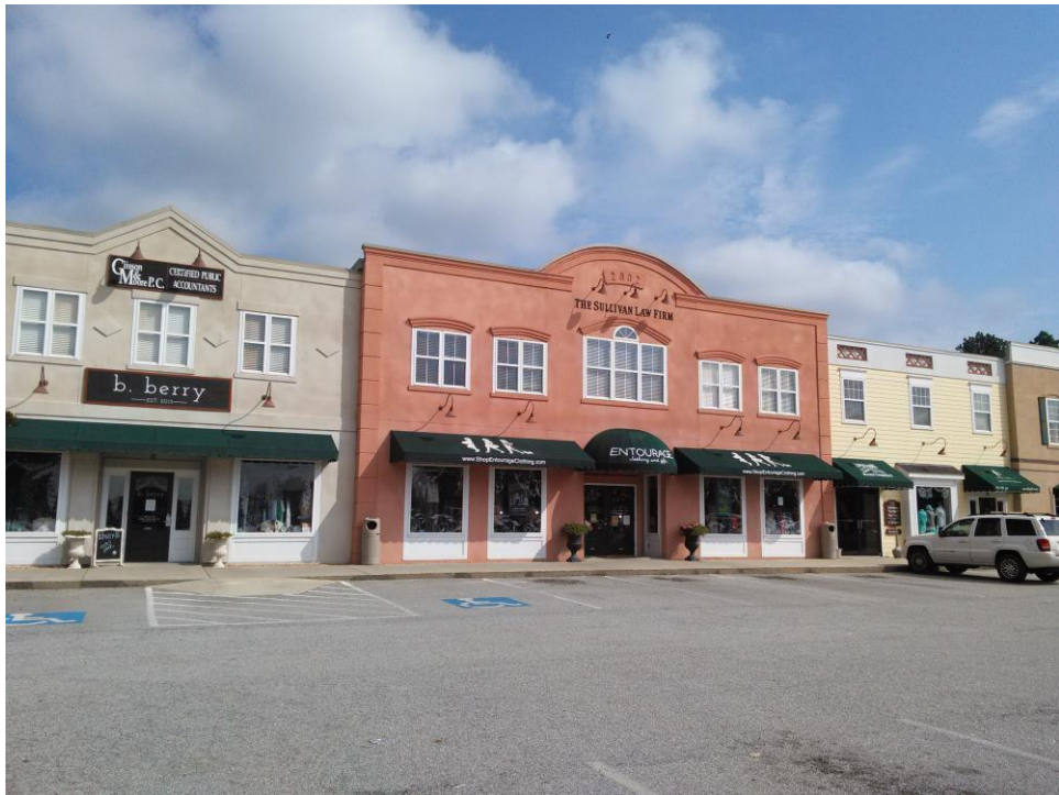
Picture 8: Wall Signs Installed at Adjacent Properties
