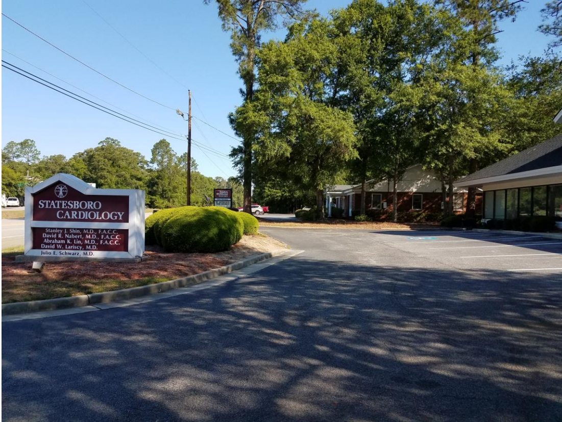
Picture 1 Proposed Location Depicting Parking Lot facing North
