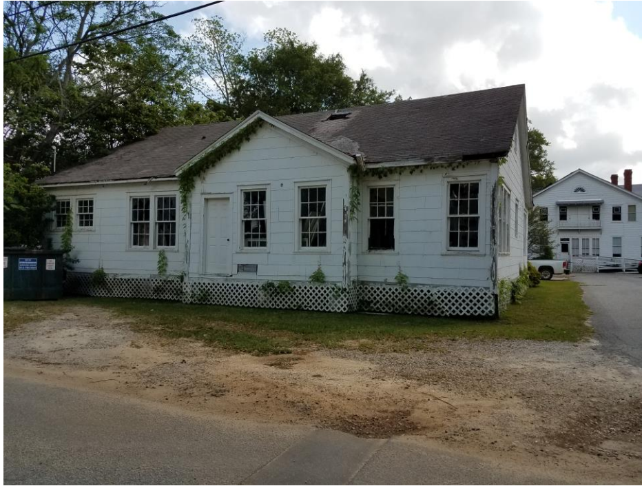
Picture 6 Adjacent Property East of Subject Site
