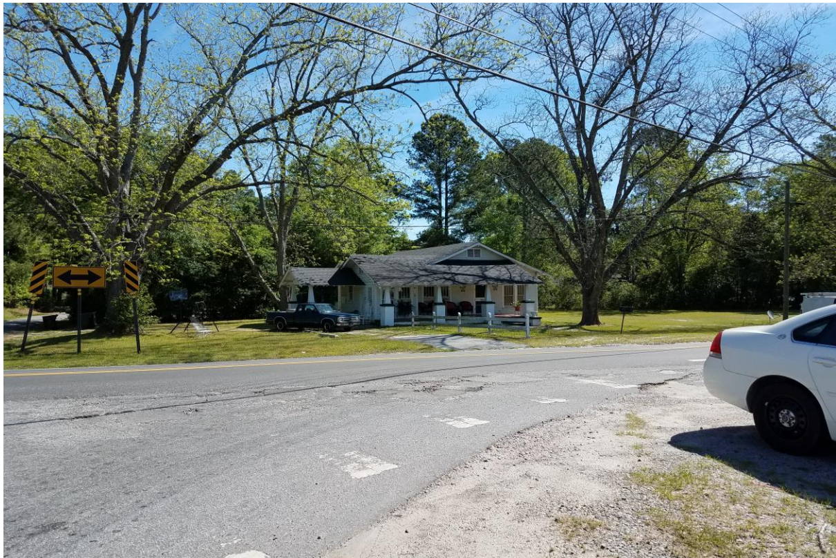
Picture 6 Single-Family Dwelling Unit on West Parrish Street Zoned R3 (Medium Density Multiple Family Residential District)
