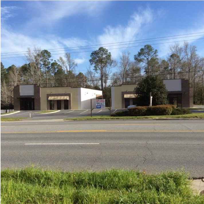
Picture 1: Front View of Subject Site Facing Northeast from Across Highway 80 East
