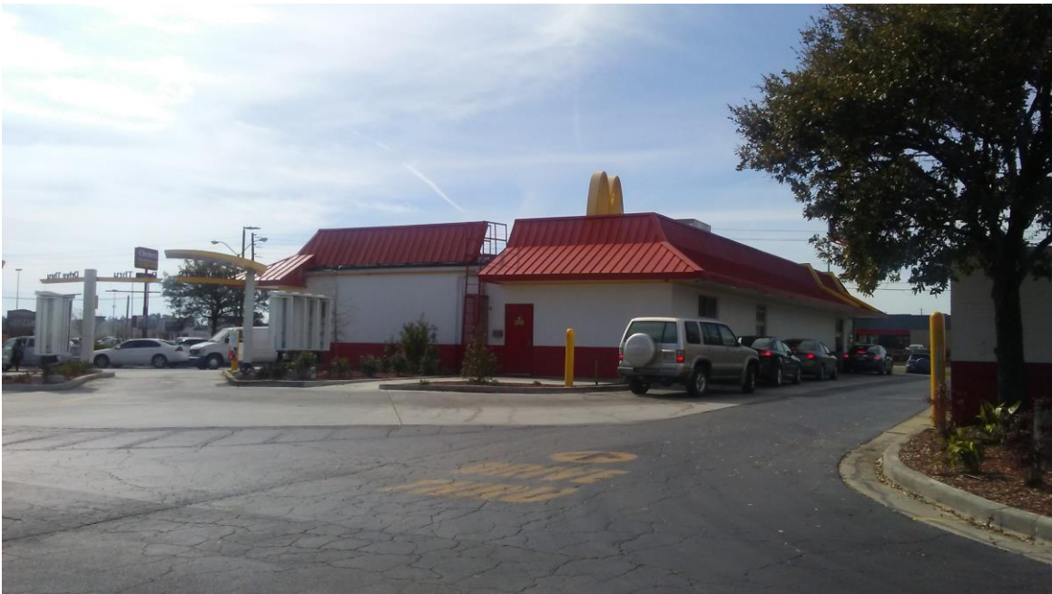
Picture 6 Rear Elevation of Subject Site
