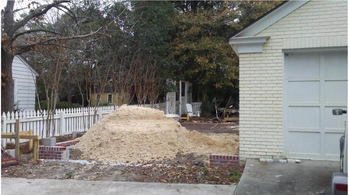
Picture 1 Subject Site Depicting Location of Carport Compared to Adjacent Property Line and Fencing
