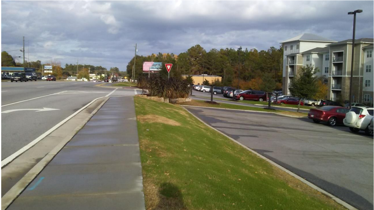
Picture 1 Approximate Proposed Location of Monument Sign (in background near yield sign) in Background Facing Northeast on South Main Street
