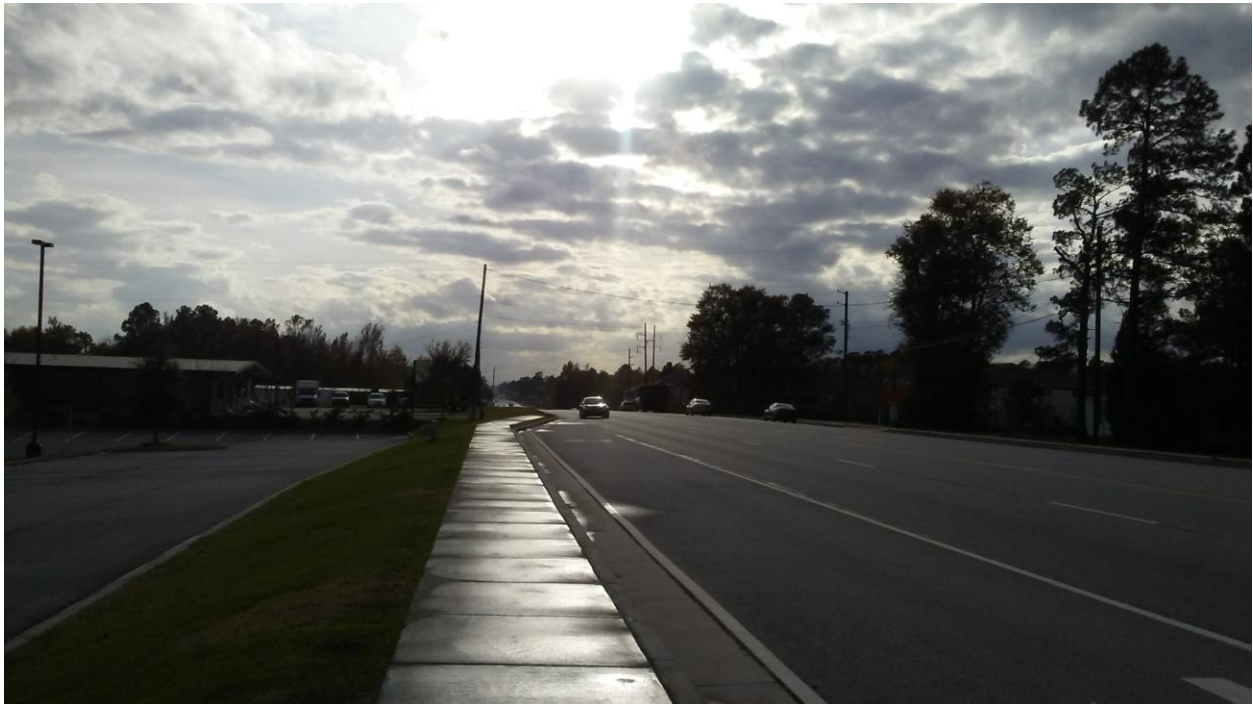
Picture 2 South Main Street Facing Northwest Depicting Potential for Traffic Approaching Proposed Sign
