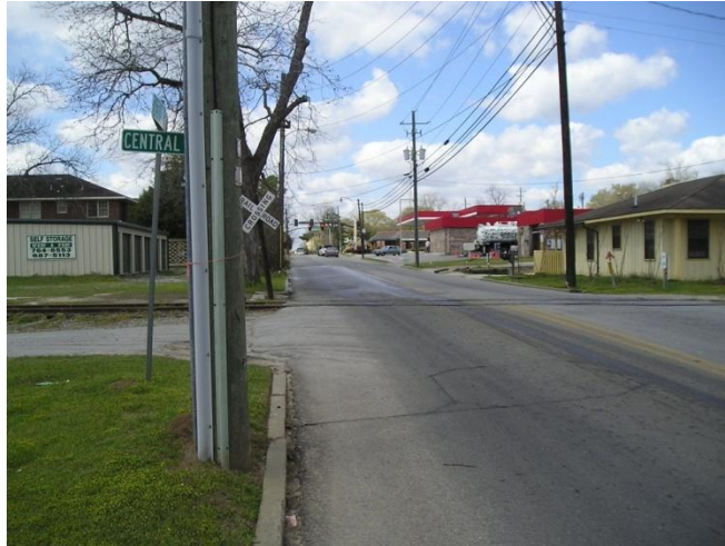
Figure 6.E.3 E. Jones Avenue Rail Crossing
