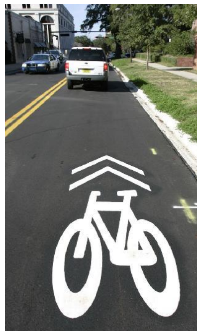
Figure 6.G.1 Bike / Ped Shared Lane Markings
